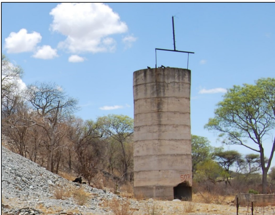
Figure 4.1 The Deblin Copper Mine concrete-lined circular shaft, grid reference 758551 mE, 7814737 mN.
