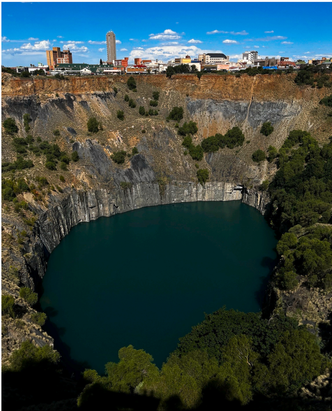
Fig. 14 a. The Kimberley kimberlite (or Big Hole), Kimberley cluster, with an original surface area of \sim 3.7 ha at the time of discovery. Wall rocks are Ventersdorp lavas (dated between \sim 2.7 and 2.8 Ga, Cornell et al., 2011) overlain by Phanerozoic Karoo sediments.
