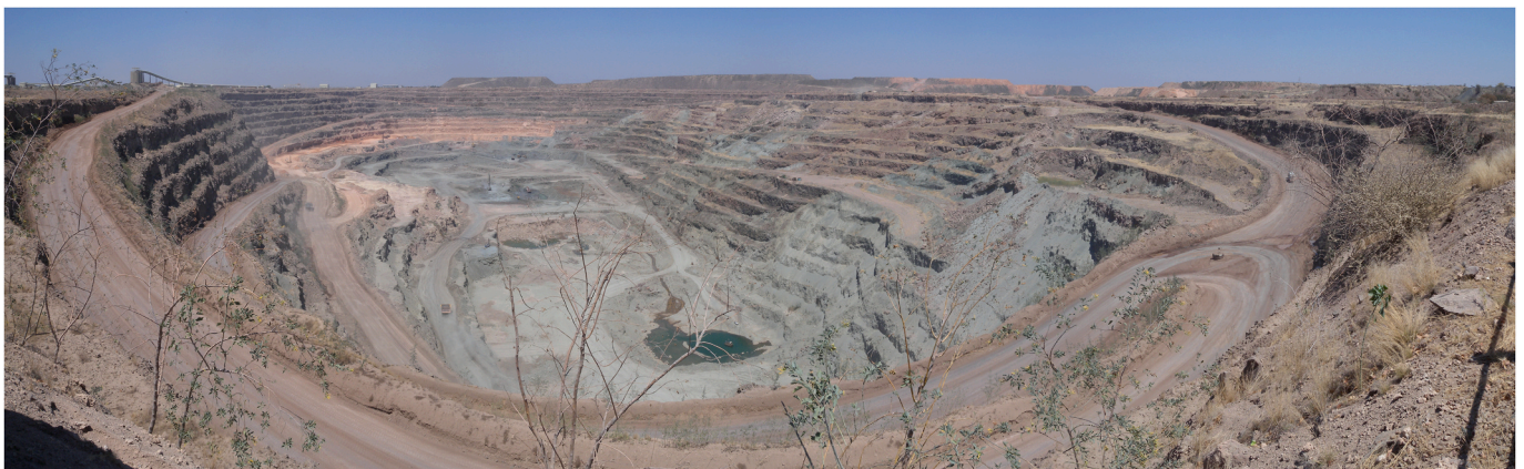
Fig. 14b. The Orapa (AK1) kimberlite, with a surface area of \sim 110 ha at the time of discovery, looking down the long axis of the pipe. Dimension of the pit is approximately 1.5 \text{ km} \times 1.0 \text{ km} (Image kindly provided by Prof. Frank Eckardt of the University of Cape Town).
