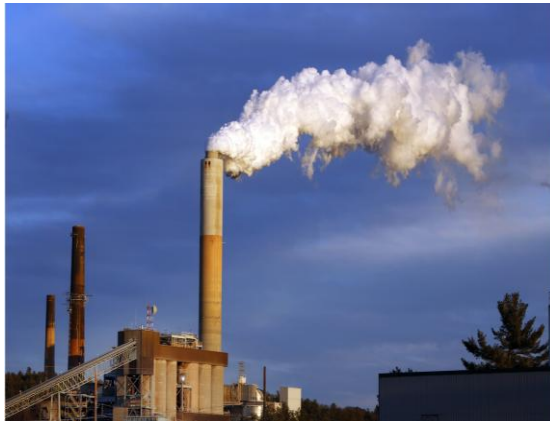
Fig 4G above shows a factory emitting smoke into the air
