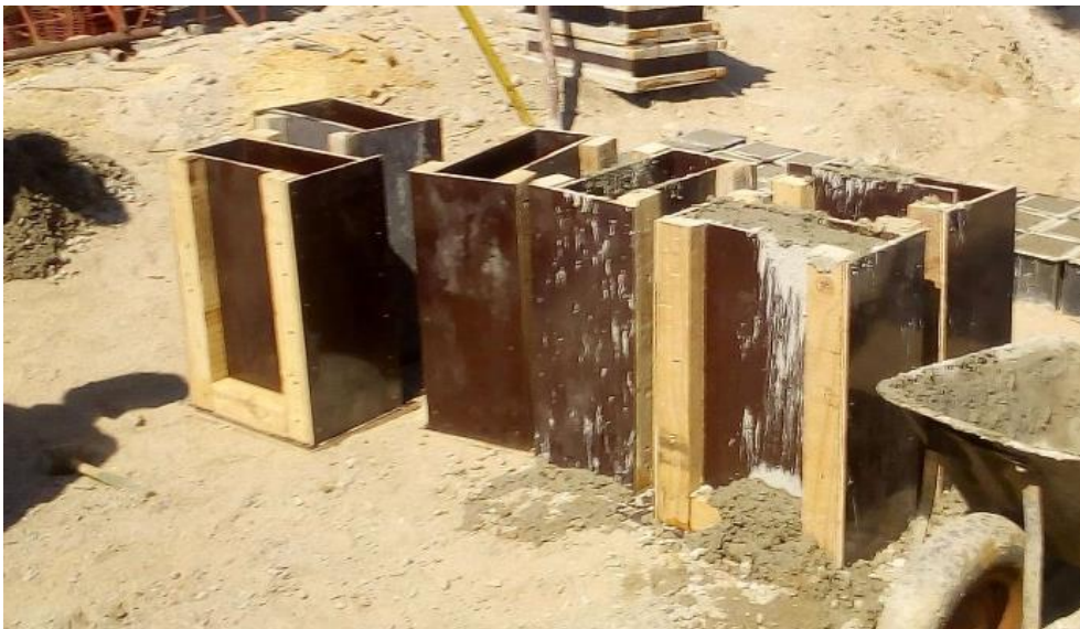
Figure 3-23 -Durability test panels representing bridge piers and abutments
