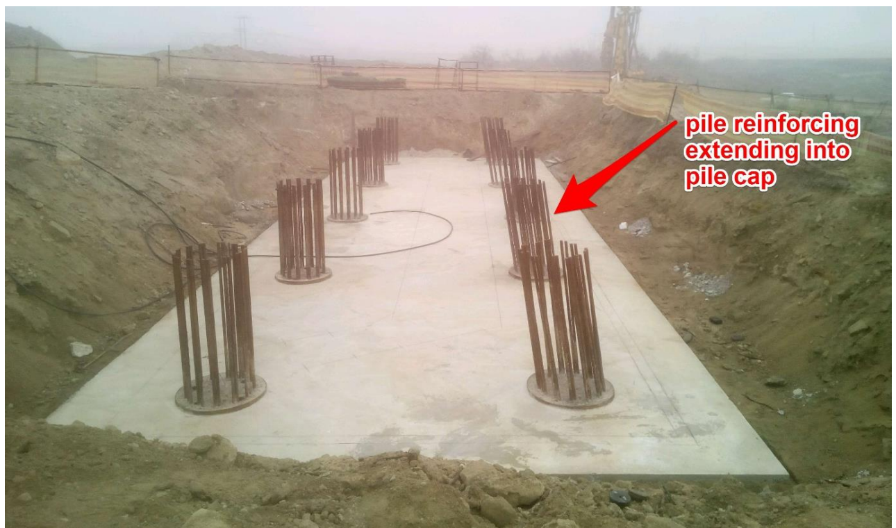
Figure 3-5 - Photograph of reinforcing steel bars extending from piles into the pile cap
