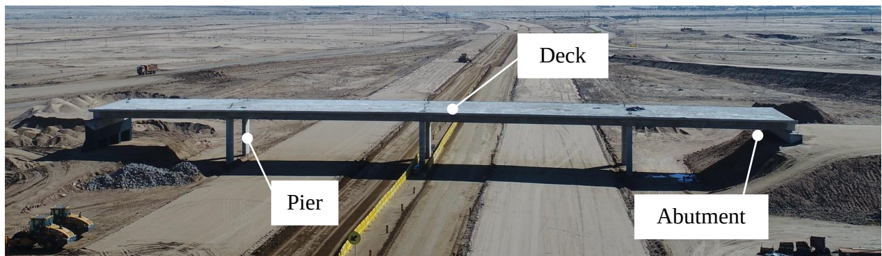
Figure 3-3 - Bridge elements
