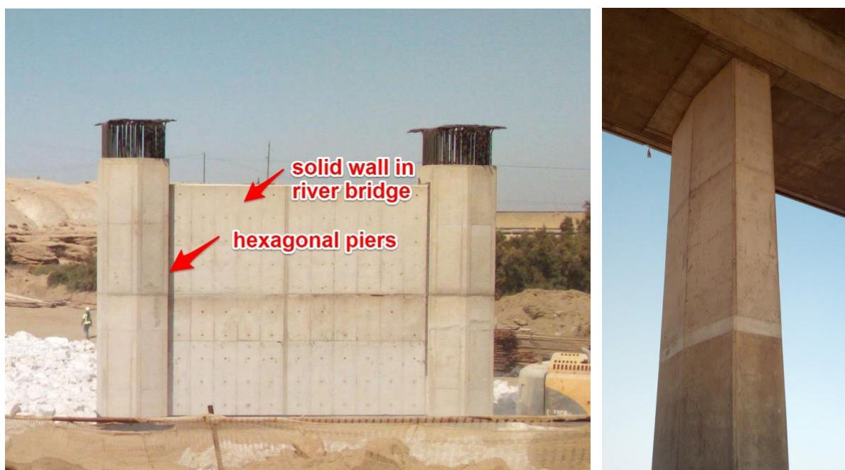
Figure 3-8 - Typical bridge piers
