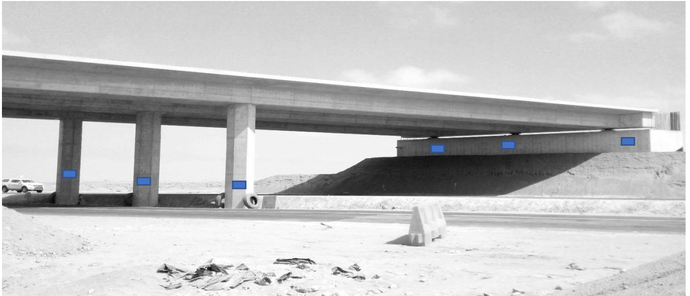
Figure 3-29 - Typical location of representative areas for cover testing on bridge substructure
