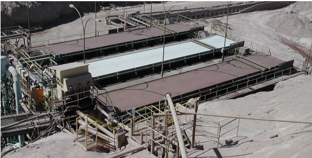
Figure 2.21: Rigid belt filters installed at an Anglo American copper mine in Chile.
