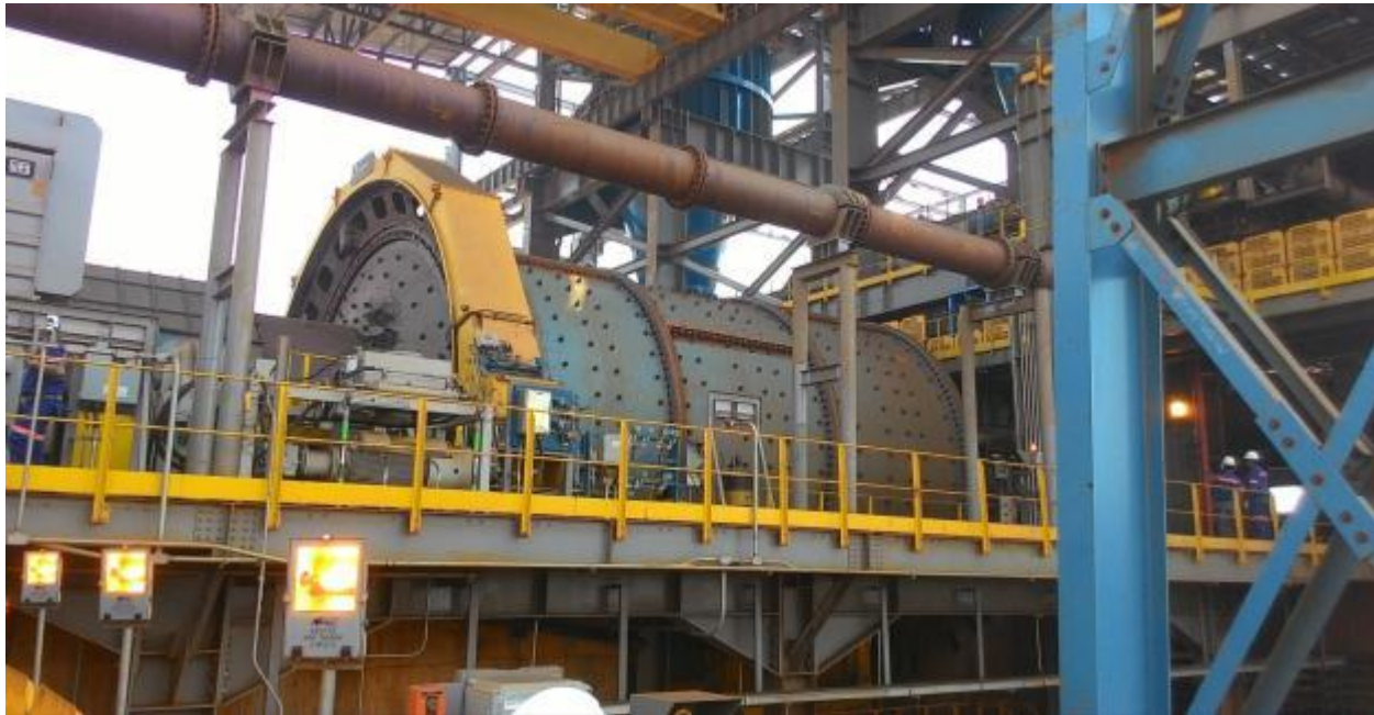
Figure 2.8: Ball mill located at the Minas-Rio operation.
