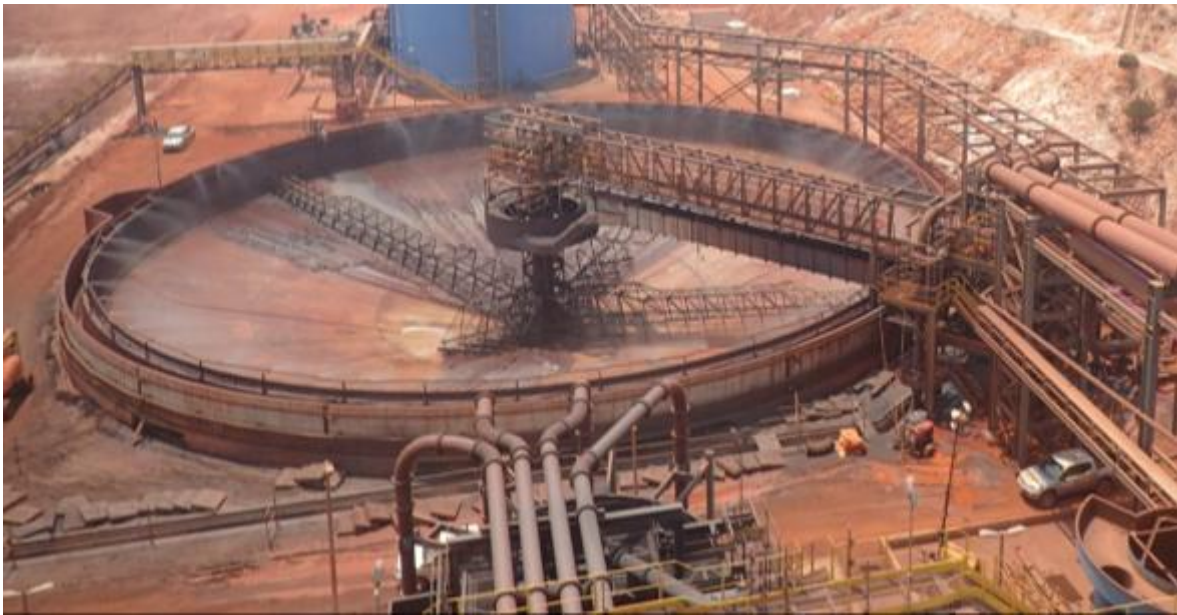
Figure 2.15: Thickener before commissioning showing feedwell and rakes at the Minas-Rio operation.
