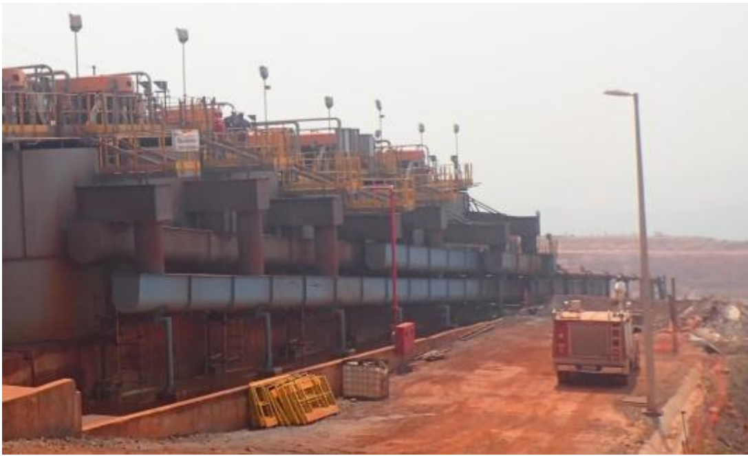
Figure 2.12: Flotation cells at the Minas-Rio operation during construction.
