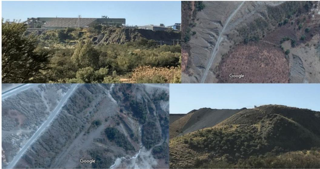
Figure 1.2 Visual representation of some eroding tailings at the Cullinan mine site.
