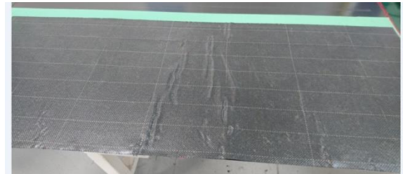
(c) Repair plies application
