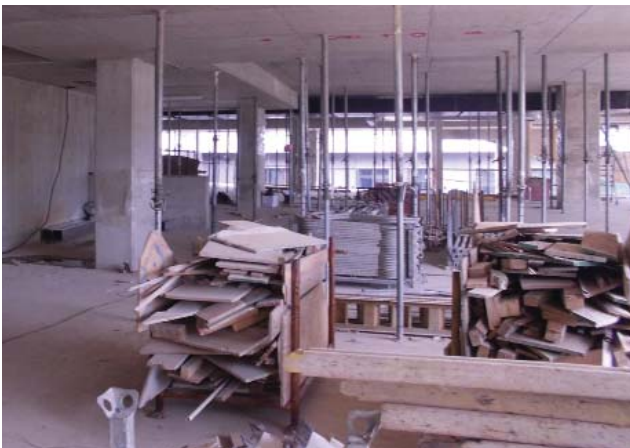
Fig 1.1: [Photograph by Author] Hoarding of construction waste on Site “X”, which is the construction of a large A-grade high rise office block in Sandton, Gauteng.
