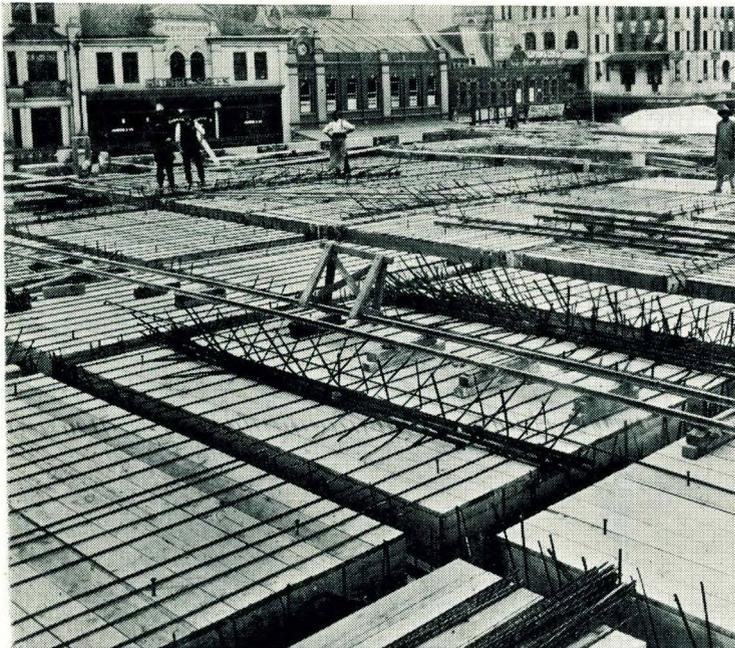
Reinforced Concrete Beams, Slabs and Columns
