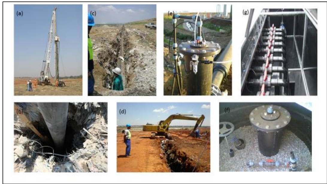
Figure 2.17: (a) Drill rig used to install vertical wells, (b) vertical well installation into drilled hole, (c) and (d) horizontal well installations, (e) knock-out pot, (f) gas well head and (g) manifold box where horizontal well heads are housed.
