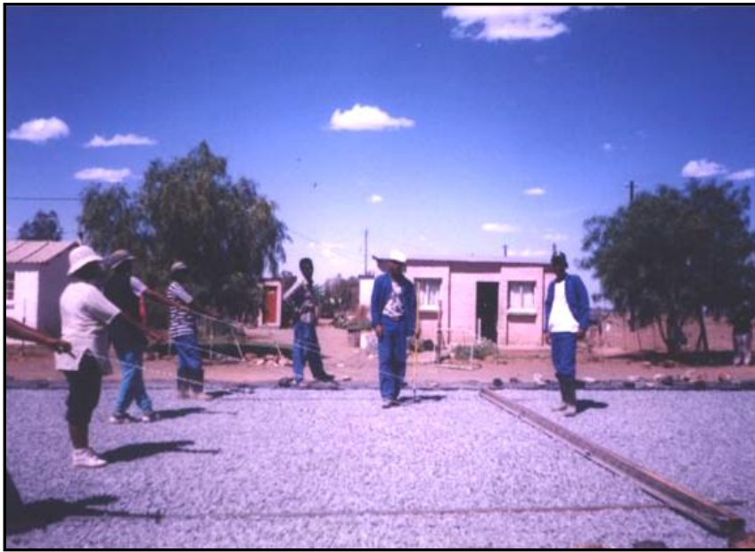
Photo 3.12: Straight-edge pulled by workers (Victoria West)
