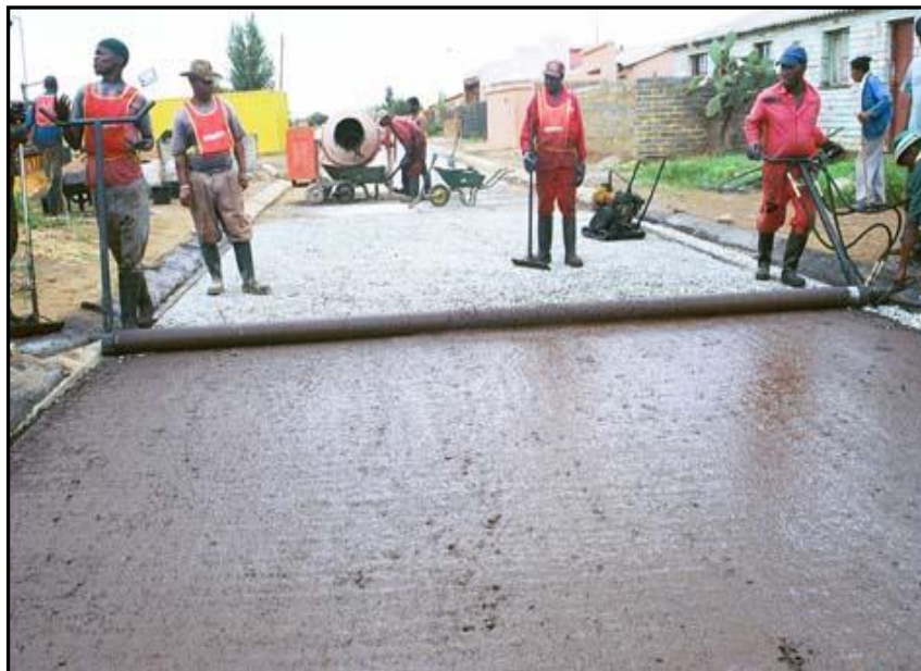
Photo 3.4: Spinning beam as final template
