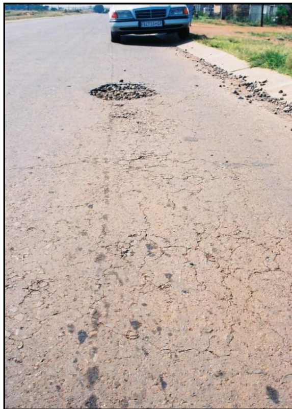
Photo 3.1: Ring road constructed with too large aggregates. Note the cracks around the stone pinnacles. Secondary distresses, ravelling and potholes also visible.
