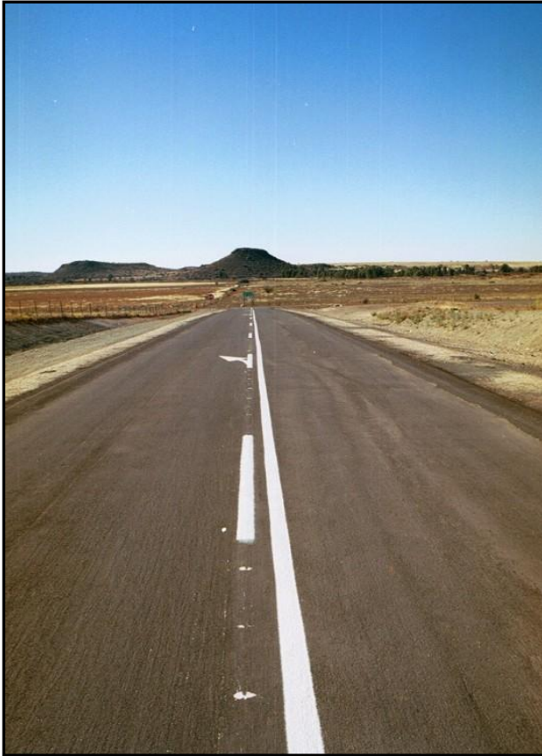
Photo 3.8: High speed cambered provincial road constructed using a Slurrybound Macadam surface (Koffiefontein/ Oppermansgronde – Free State Province)
