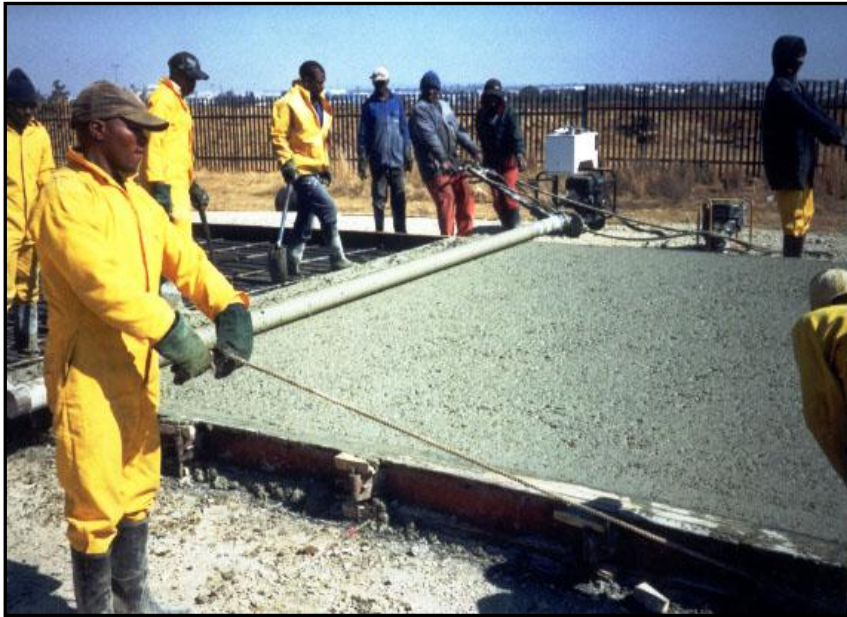
Photo 3.13: Spinning beam used with concrete inlays on the N3
