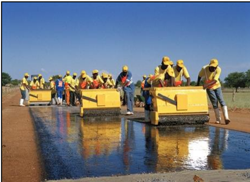
Photo 3.11: 'Chippy' a labour-intensive chip spreader
