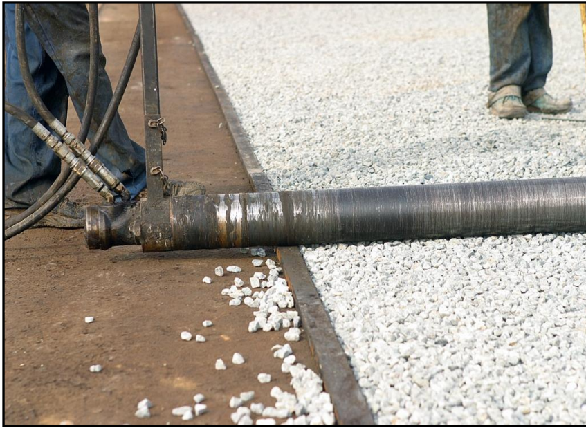
Photo 3.3: Spinning beam on guide rail
