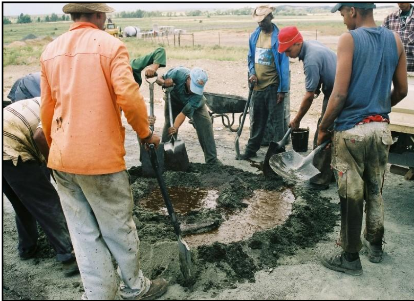
Photo 3.14: Slurry mixing by hand
