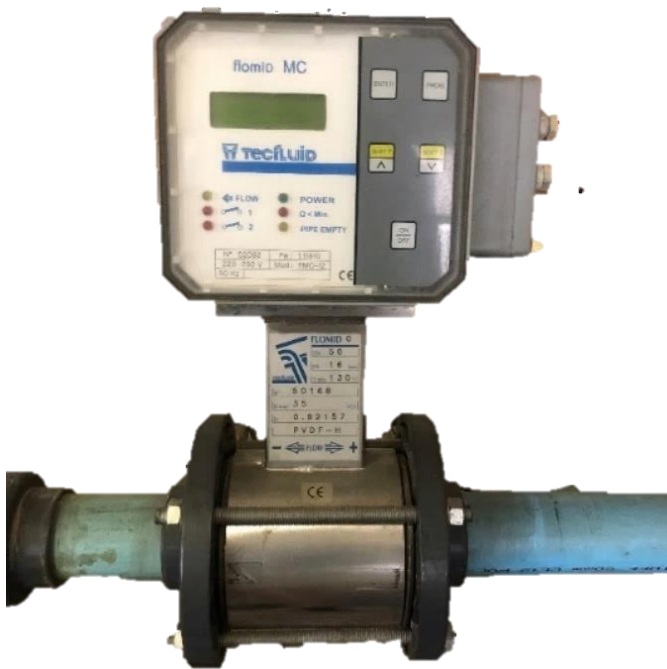
Figure 3-4- Electronic discharge gauge
