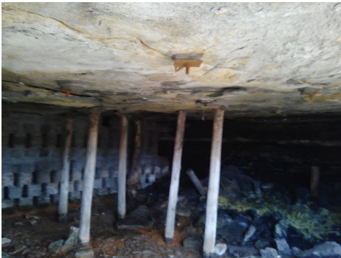
Figure 5.4. A stope completely depleted of coal and only the sandstone layer left behind. The poles are used to support the roof. This shows why there was no need to include the coal seam in the models.
