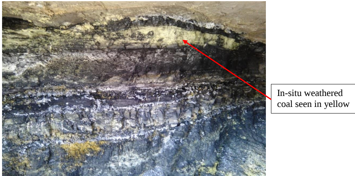
Figure 2.5. Underground tunnel opening showing a weathered coal seam and traces of pyrite and precipitated sulphur.
