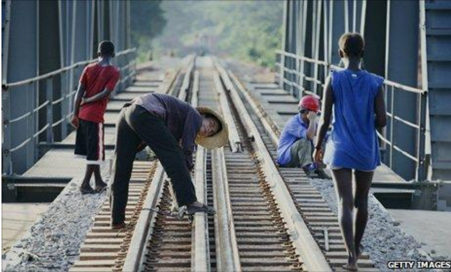
Appendix 3: Adapted from BBC News website. Part of the Benguela railway line which is being repaired.
