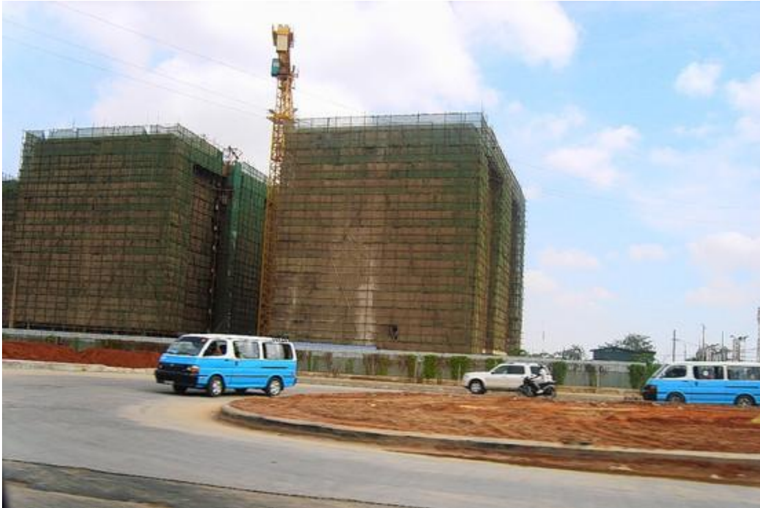
Appendix 1: Adapted from The Wall Street Journal. The Kilamba Kiaxi social housing in Luanda is being built by the Chinese.
