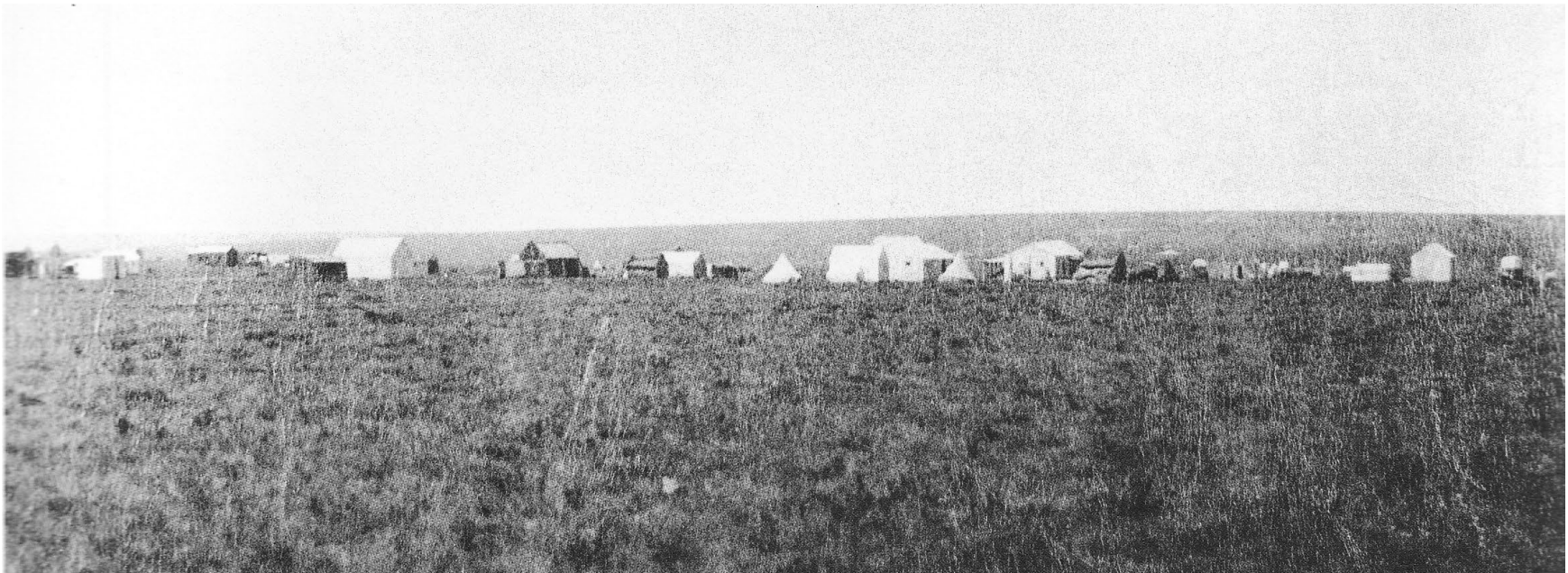
Fig 2.2 Ferreira's camp in 1886 with tent and reed structures in the veld (Johannesburg One Hundred Years)
