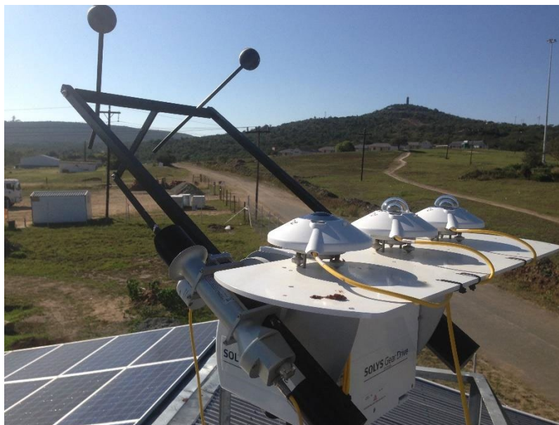
Figure 3.5: Solar radiation and weather station at the SolarWatt Park, University of Fort Hare
