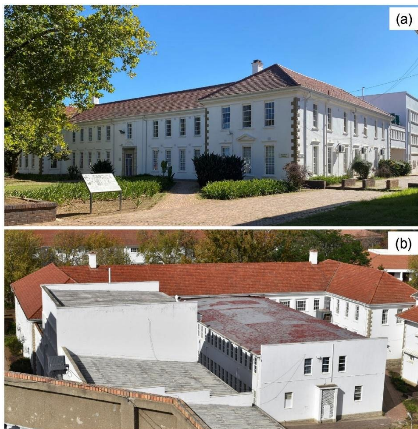
Figure 3.2: The Physics Building at the University of Fort Hare; (a) front view and (b) rear view
