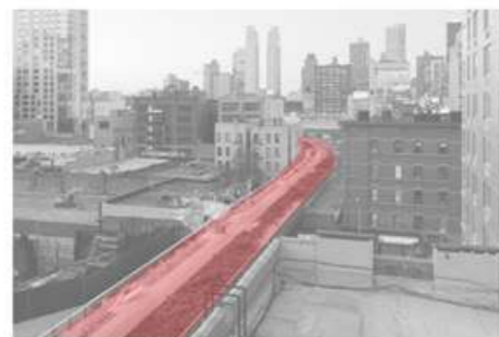
The High Line Bridge
