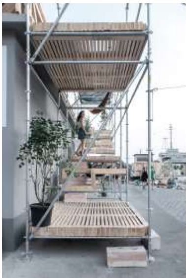
Figure 221: Scaffold stair and deck in Rijeka (Dezeen Palagani, 2019)
