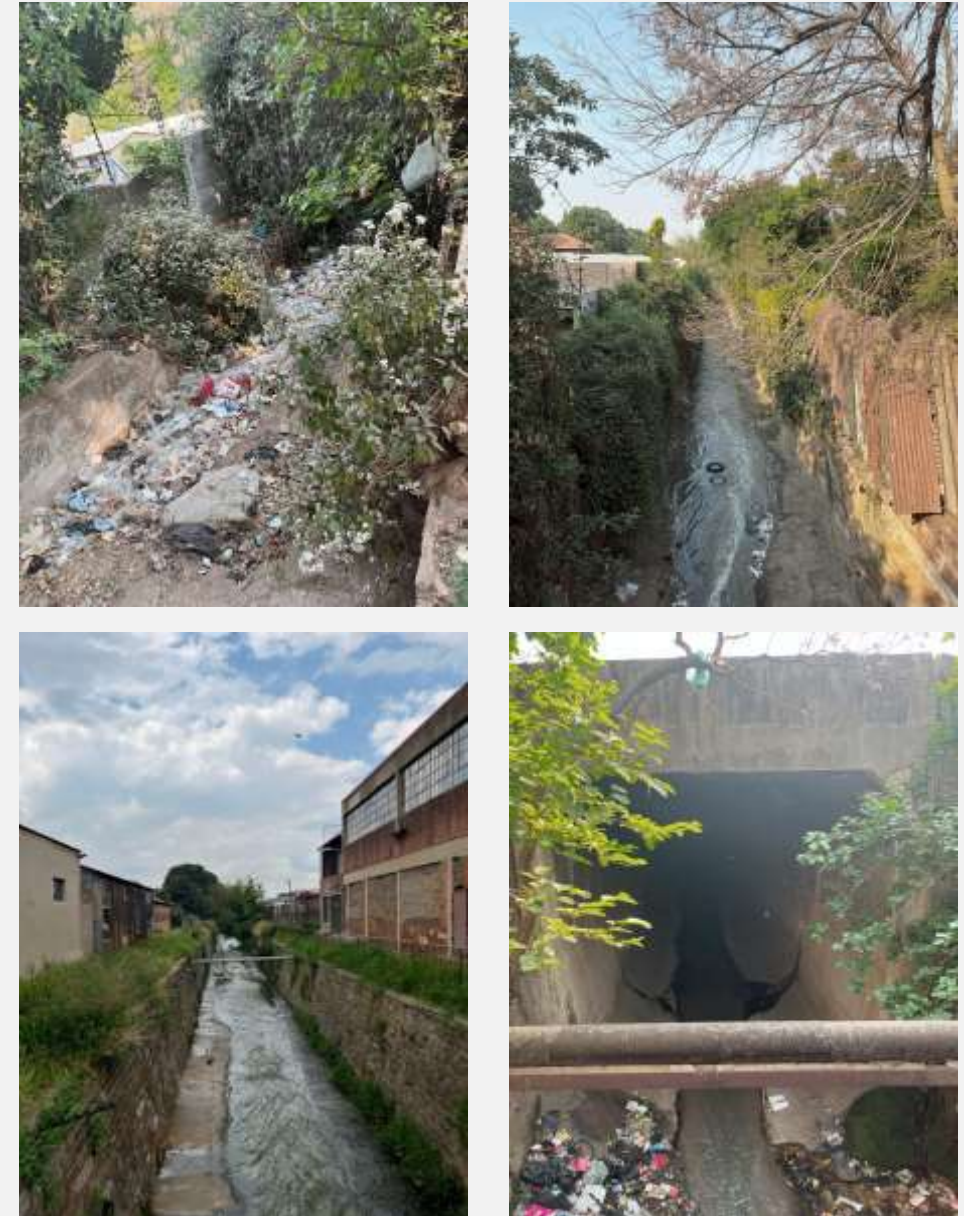
Figure 67: The river flowing through the valley, choked with litter and plastic, the stench of industrial waste and sewerage always present (Photos by author)
