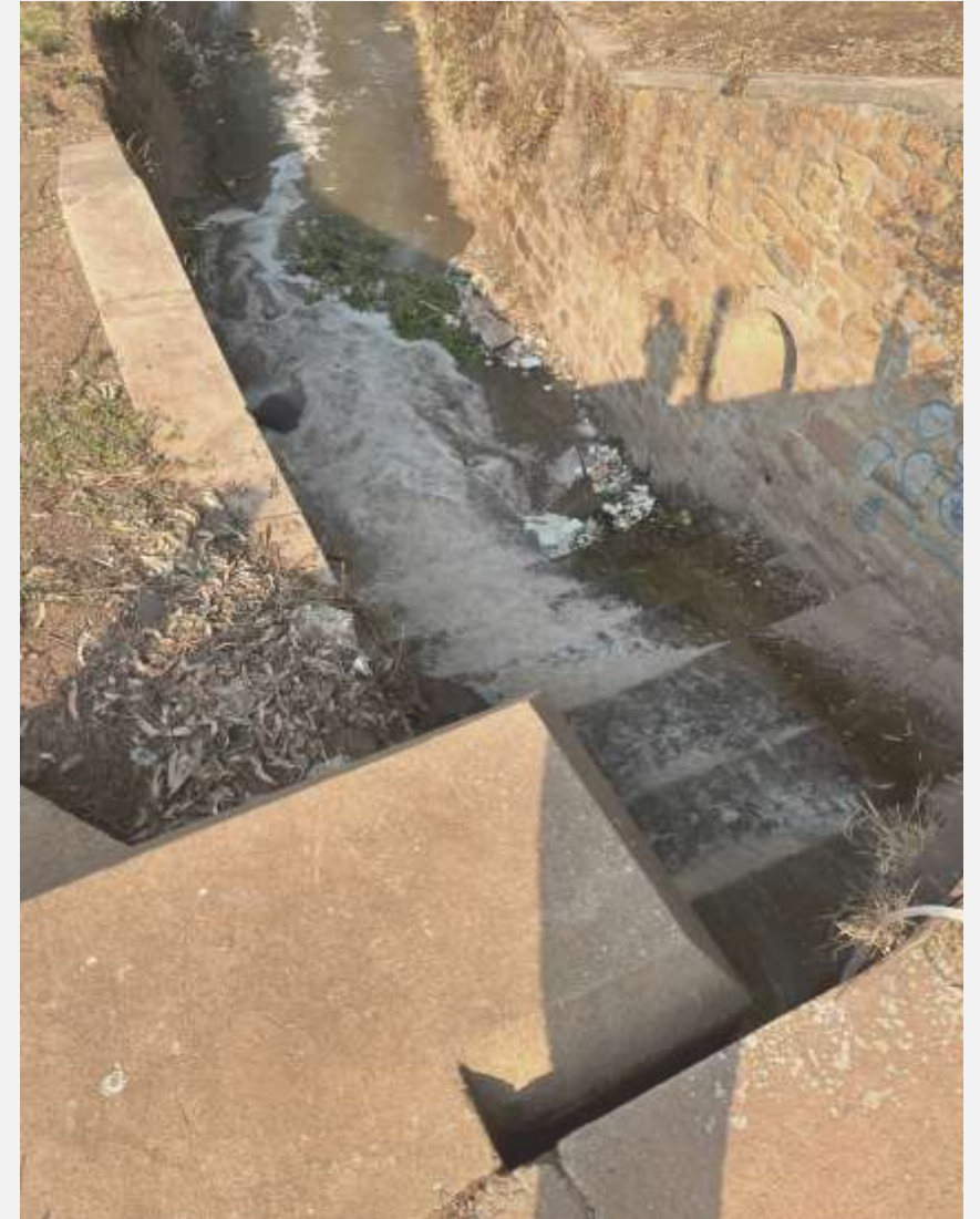
Figure 4: Jukskei River flowing in a stone channel (Photo by author)
