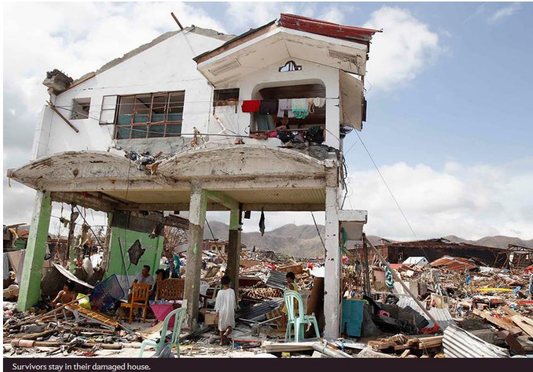
Figure 1.3: Damaged house after Super Typhoon Haiyan (Jaramillo, 2013).
