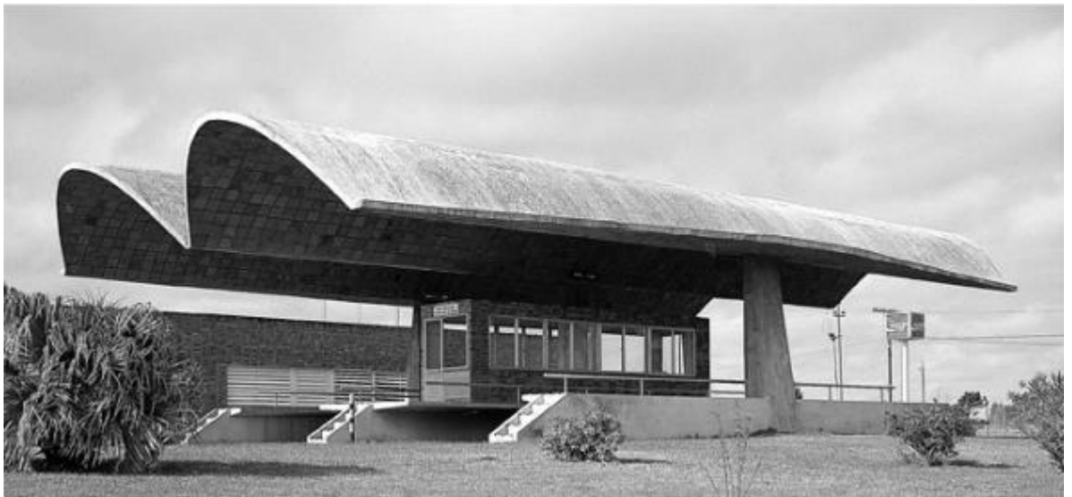
Figure 2.21: Double cantilever free-standing vault at Refresco del Norte, Uruguay (Pedreschi, 2006).
