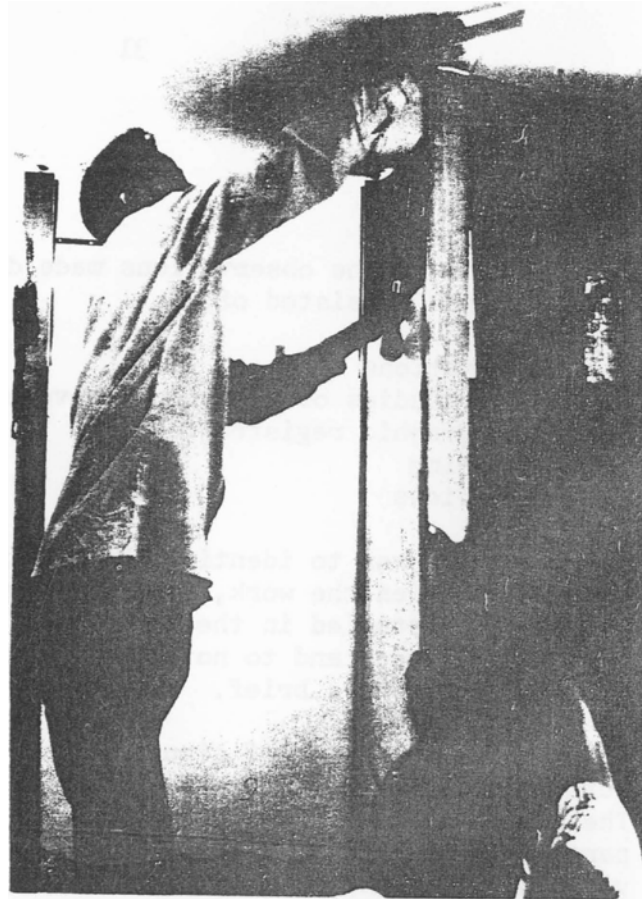
...mounting the partitions for an observer's cubicle.
