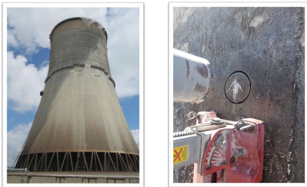
Figure 0-1 - Overall image of CT 245B and the core drilling rig being aligned into place
