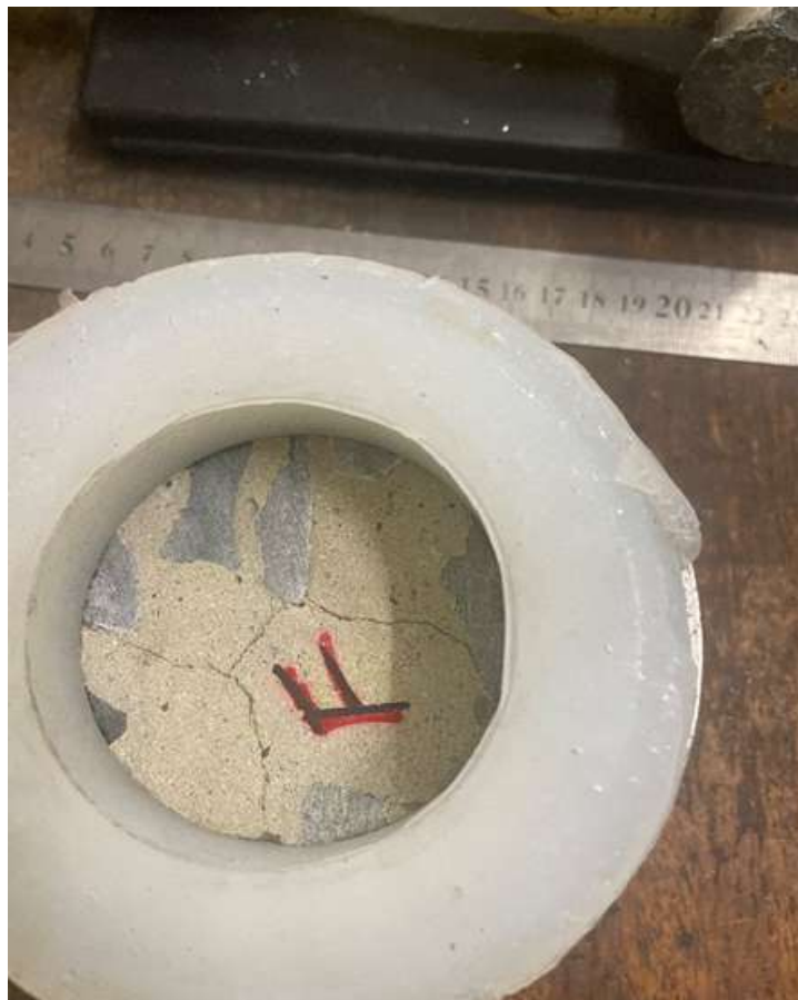
Figure 3-19: Cracked specimen inside the collar rig.
