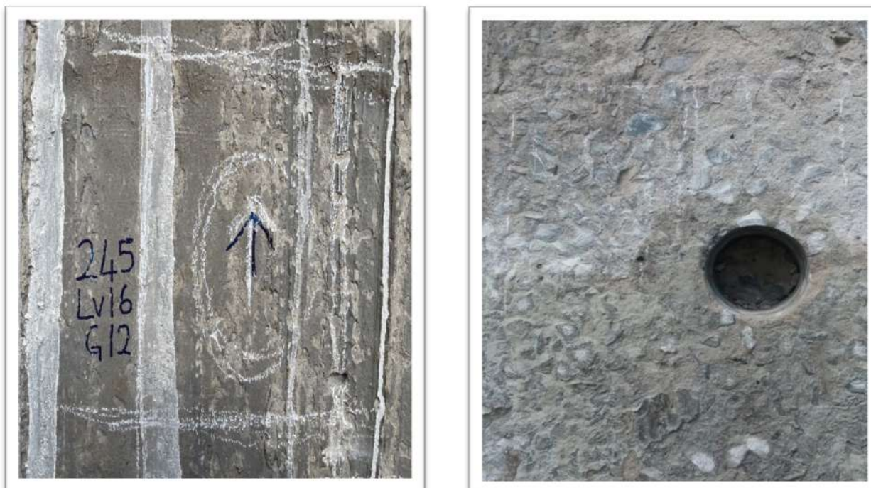
Figure 0-2 Marking out of core location and after core was extracted
