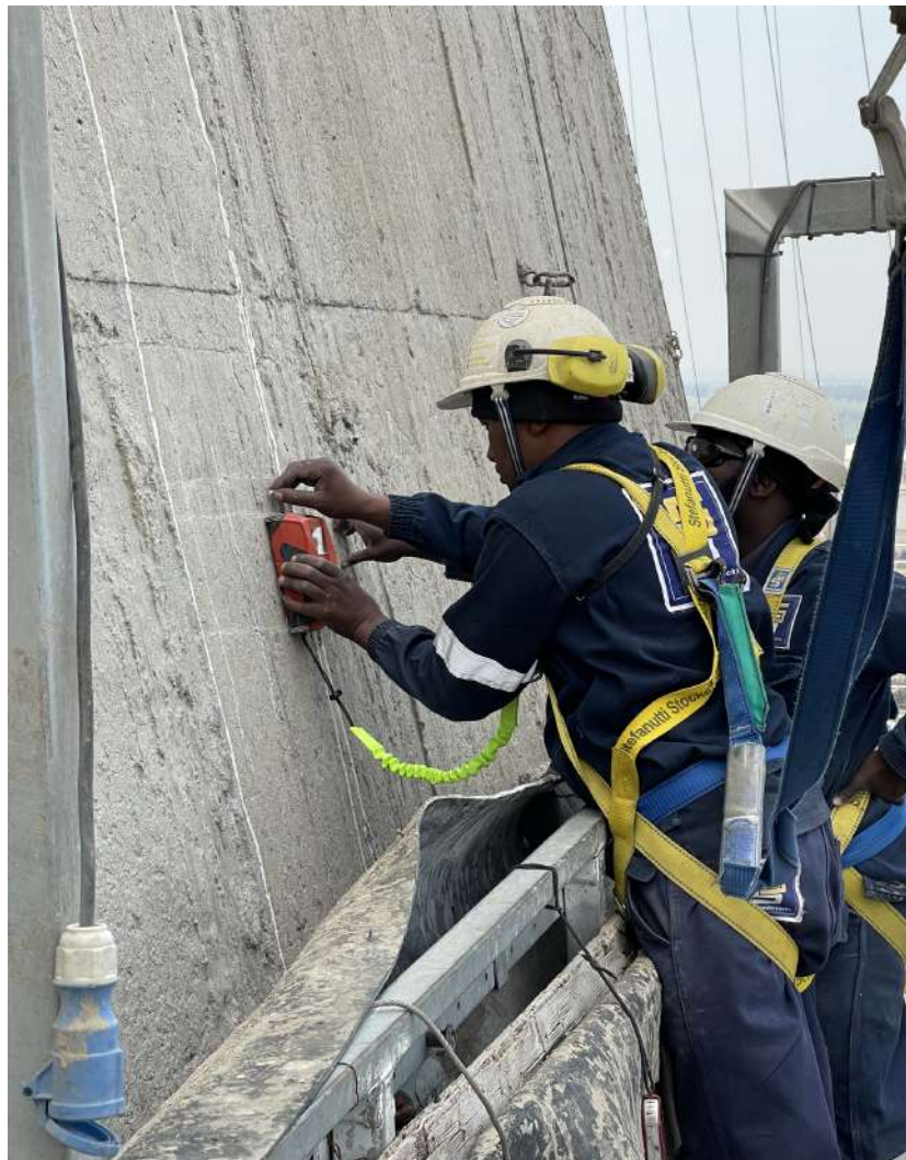
Figure 3-8: Contractor using GPR Technology to identify the location of Reinforcing bars.
