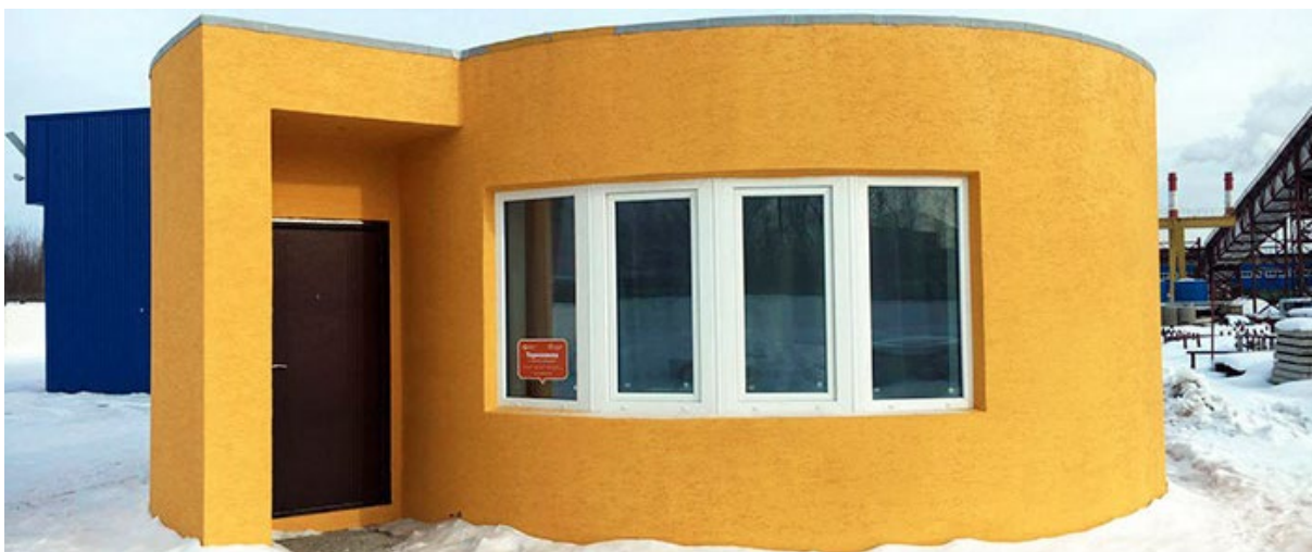
FIGURE 4: THE COMPLETED 3D PRINTED HOUSE BUILT IN 24 HOURS BY APIS CORE, 2017.
