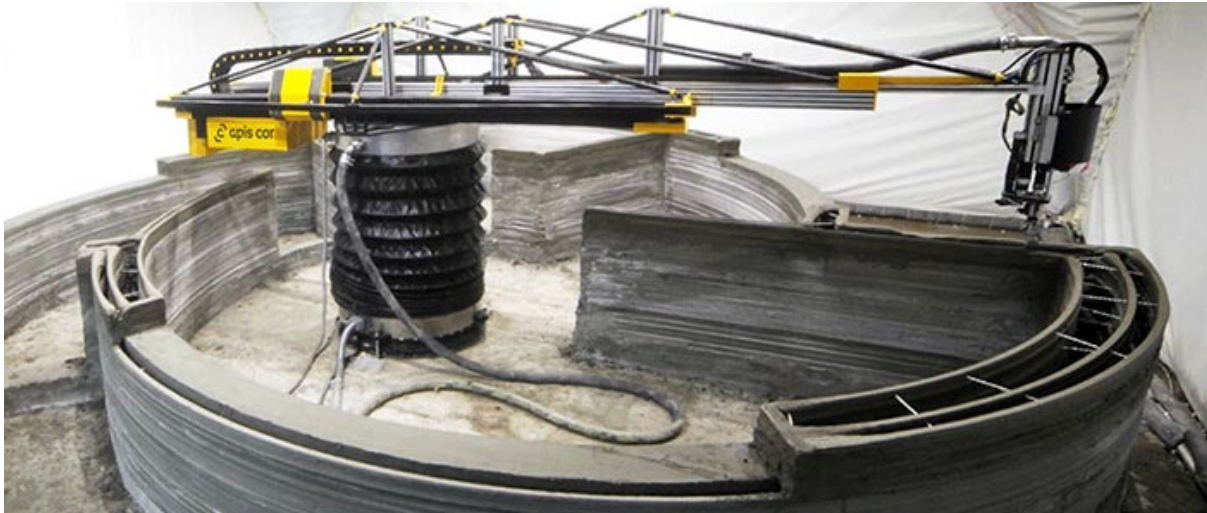
FIGURE 3: A MOBILE CONSTRUCTION 3D PRINTER IN THE PROCESS OF PRINTING A HOUSE BY APIS COR, 2017.
