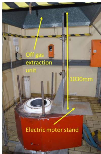
Figure A6: Electric motor stand on the furnace shell
