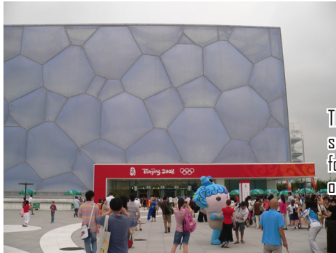
AQUATIC CENTRE PWV architects( Beijing 2008)
