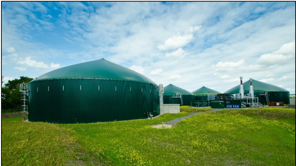
Figure 2.1: Anaerobic digesters at a biogas plant (Shutterstock Images, 2018)
