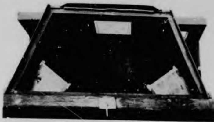
Fig. 18. An inside view of the box with a picture inserted in the back frame. The top has been removed.
