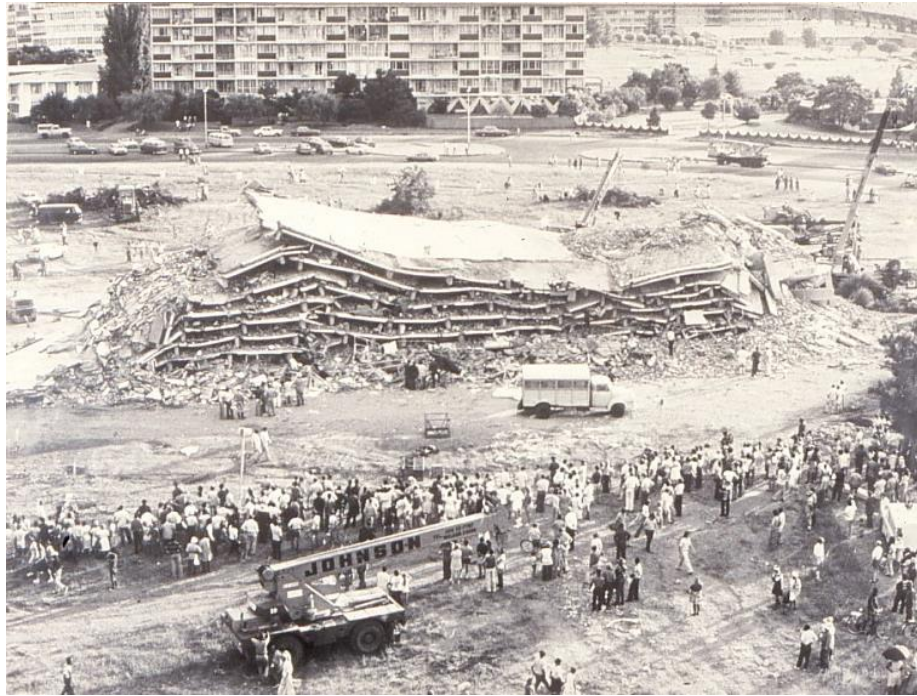
Figure 2.13 Damage to a multi-storey building during M_L 5.2 seismic event in Welkom area, Durrheim et al. (2006)
