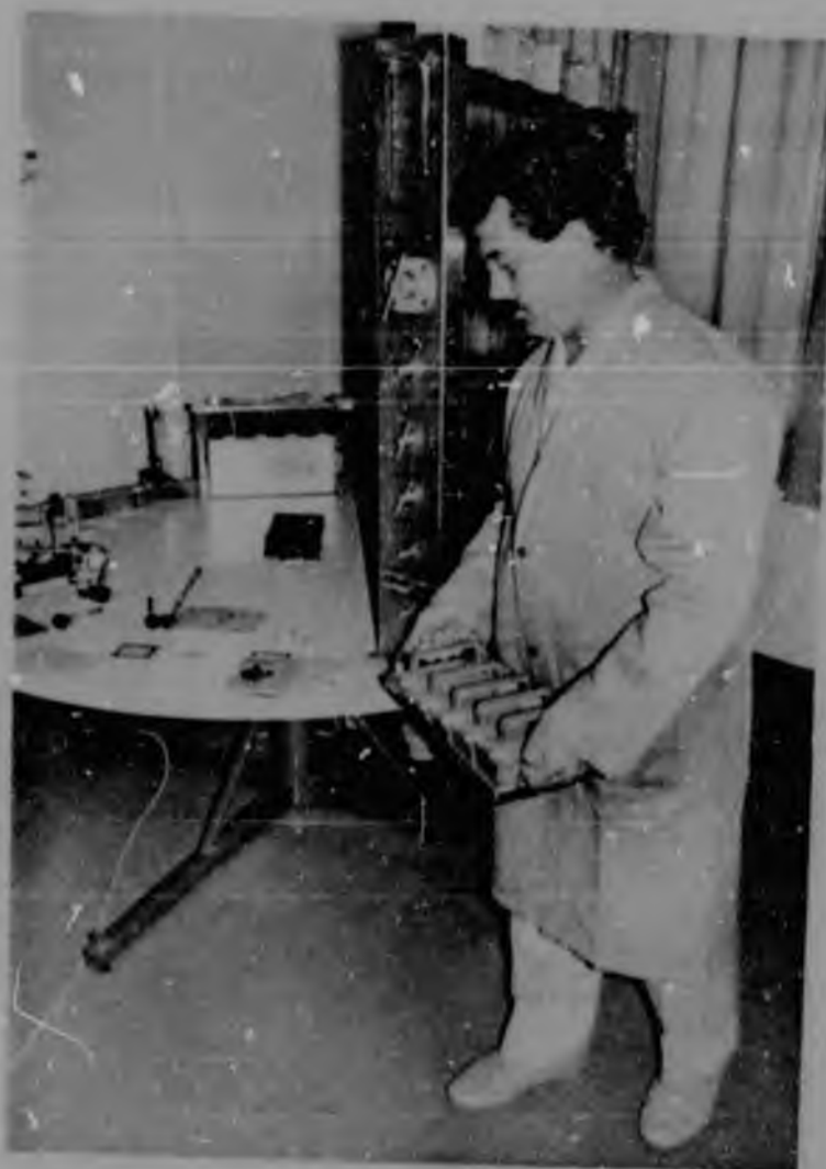
Figure 69 Test 73 showing the testee carrying a 13,59 kg (30 lb) tray of weights past the console on his 10 m journey around the table. Test 72 is similar, carrying a 3,62 kg (8 lb) weight in one hand.
