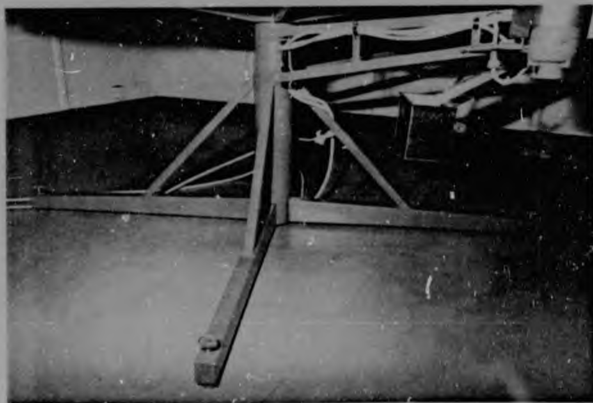
Figure 15 Central pillar on which the table top revolved. Note the splayed legs for stability.
