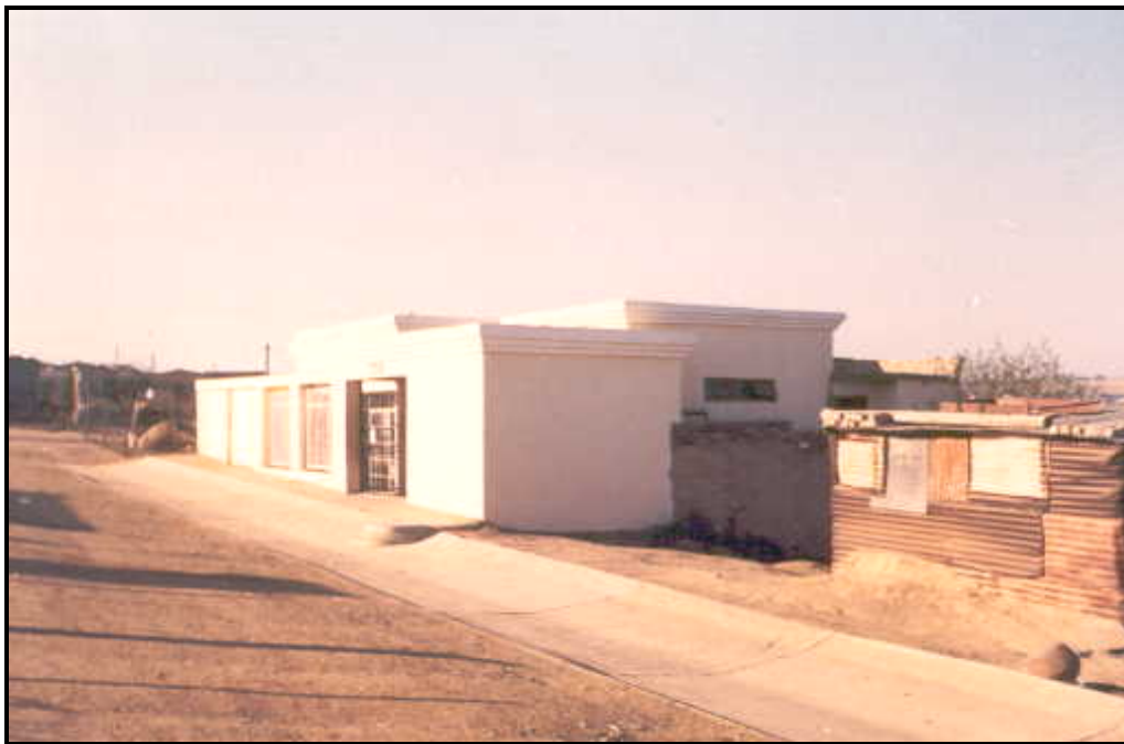
Photo 6.8. A seven roomed house next to a shacks on a site and service site in Diepsloot
