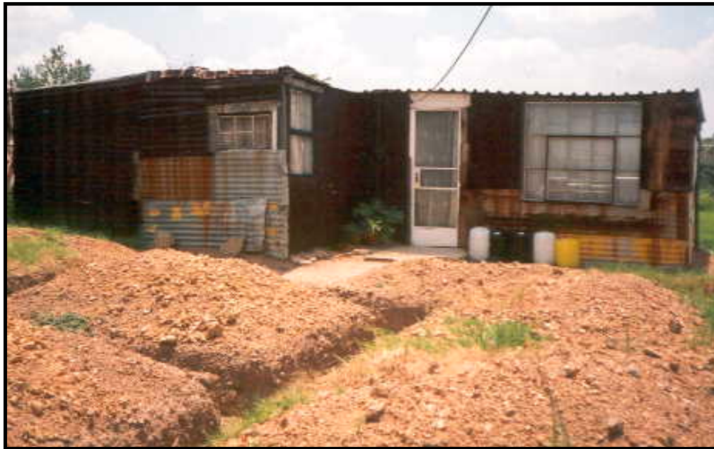
Photo 6.9. Shack with foundation awaiting top-up subsidy in Diepsloot.
