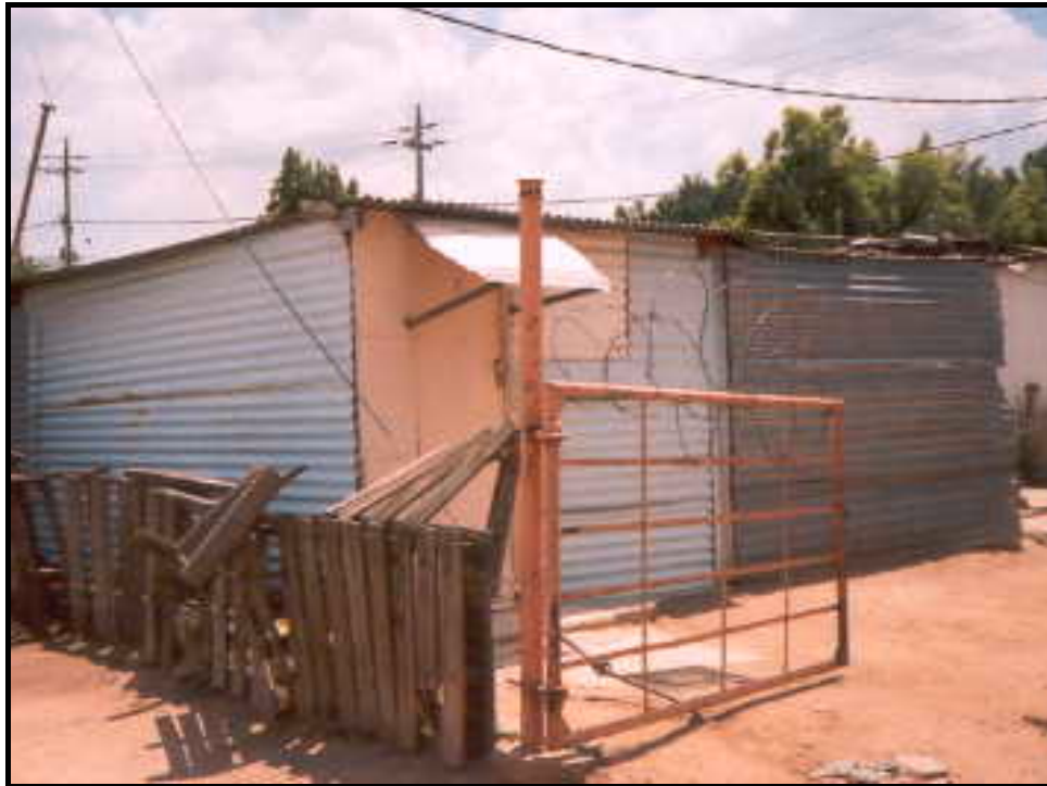
Photo 6.6. Ms Khoza's shack in the site and service area of Diepsloot
