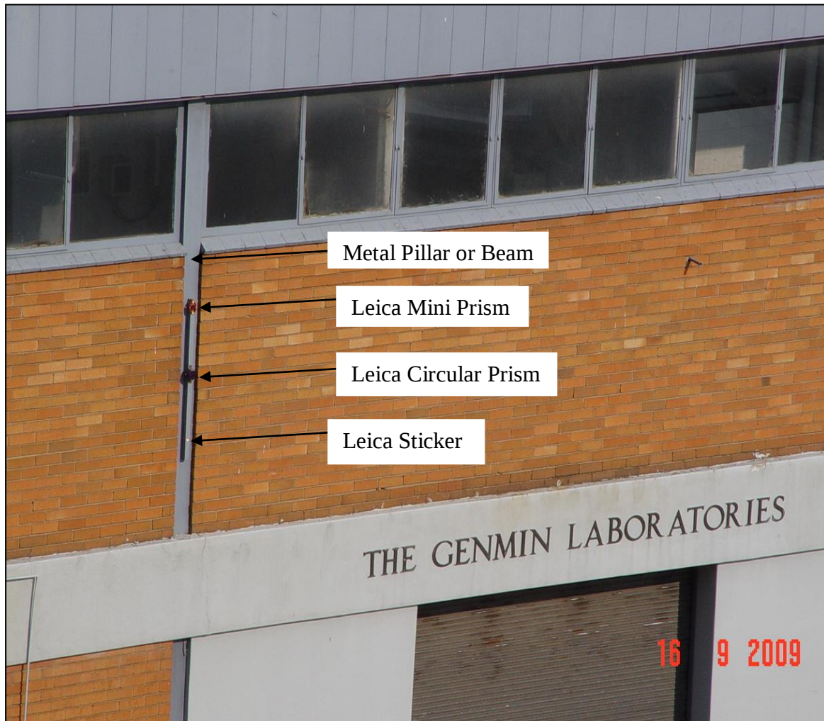
Figure 4.14: Target attached to Genmin Laboratories metal pillar
