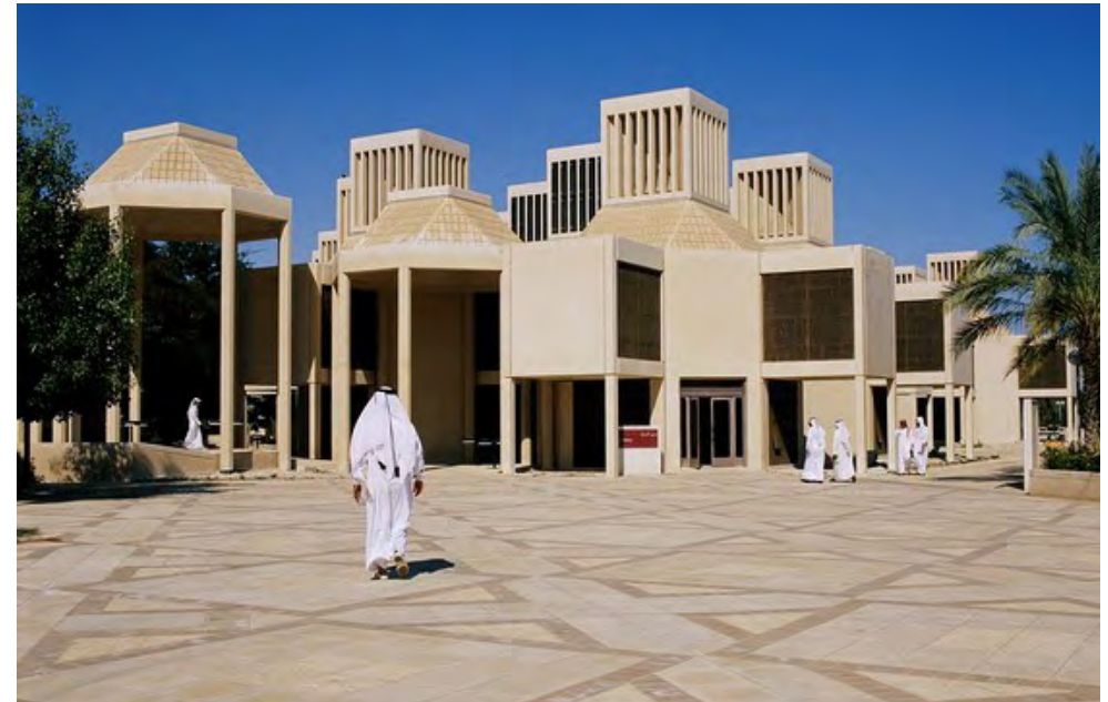
Figure 35: Dysfunctional light scoops adorn classroom roofs, University of Qatar ( www.best-masters.com/ )
