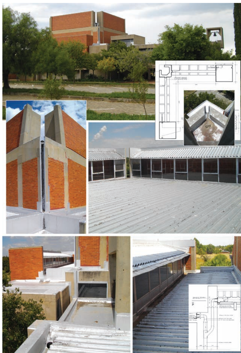
16 NGK Welkom-Wes. Seating in nave and gallery with construction details (Uytenbogaardt Papers). 17 Drainage details, NGK Welkom-Wes. Clockwise from top left: General view from north-east; Plan detail of a recessed open corner channel (Uytenbogaardt Papers); Square roof of two auditorium corner columns shaped as a sump; Clerestory monitors to auditorium roof; Clerestory monitor on a side gallery showing bend to the box gutter; Details of built-in stormwater pipes (Uytenbogaardt Papers); View from the roof of the oppersaal towards the monitor of the eastern gallery showing various waterproofing attempts; Drainage by way of recessed open corner channels on the exterior of the auditorium.
