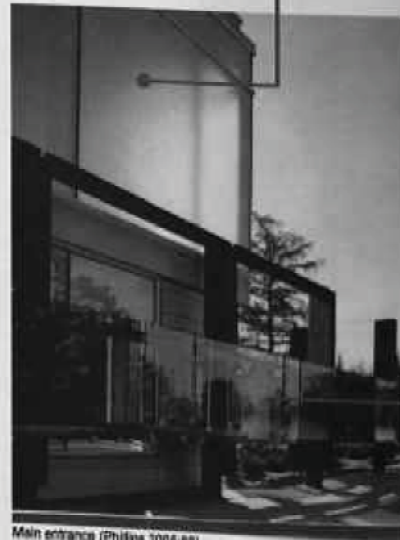
Main entrance (Phillips, 2005:68)
