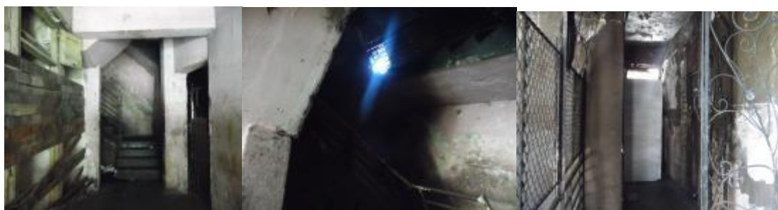
Figure 9 Shaka House foyer, corridors and ceiling
