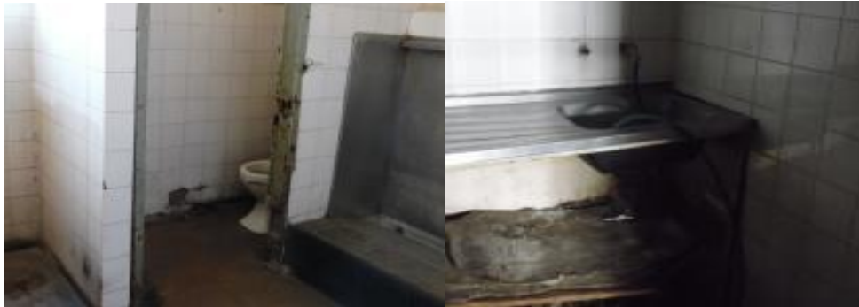
Figure 19 The locked toilet on 8 th floor and kitchen used to collect water on 8 th floor
