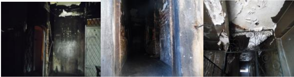
Figure 11 Shaka House corridors, walls and ceiling
