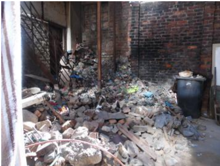
Figure 17 Rubble behind Shaka House
