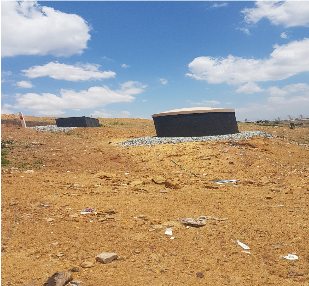
The above picture shows a landfill gas project in the City of Johannesburg
