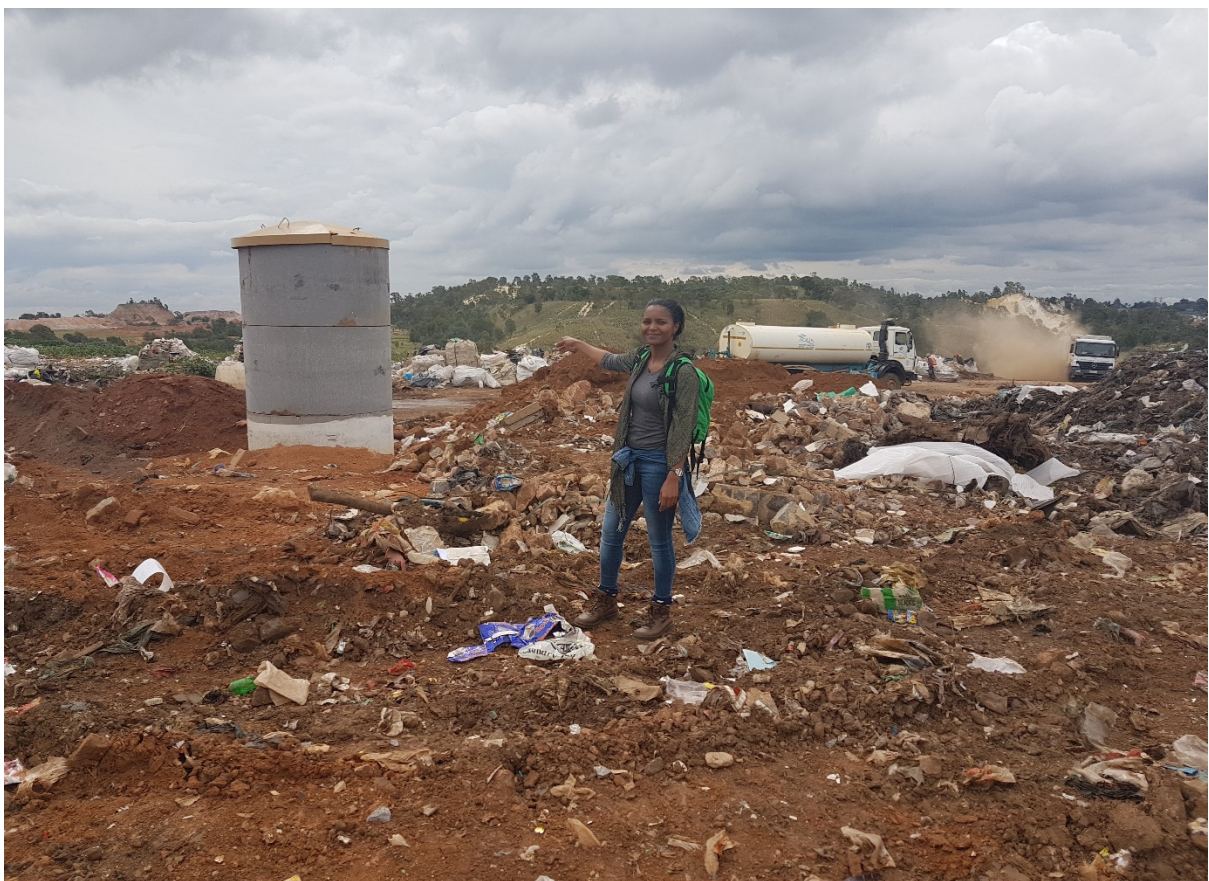
The above picture shows a landfill gas project in the City of Johannesburg
