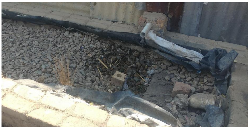
Figure 21: Inlet region of constructed wetland 1 showing large PVC elbow from inlet drain on the right. Photo taken on 23.09.2020 which was the second week of sampling after the national COVID-19 lockdown in South Africa, and therefore the vegetation in the constructed wetland had not yet grown back. (Coordinates: 26°05'17.0"S 28°06'25.3"E)
