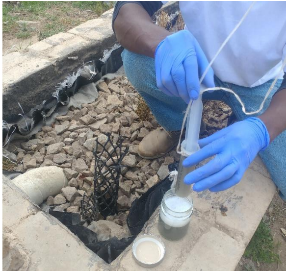
Figure 23: Inlet region of constructed wetland 2. To the left is the large white PVC elbow that connects the incoming drain to the wetland, and in the centre is the black 'cylindrical trellis' used to access inlet water in the wetland. (Coordinates: 26°05'16.1"S 28°06'25.9"E)
