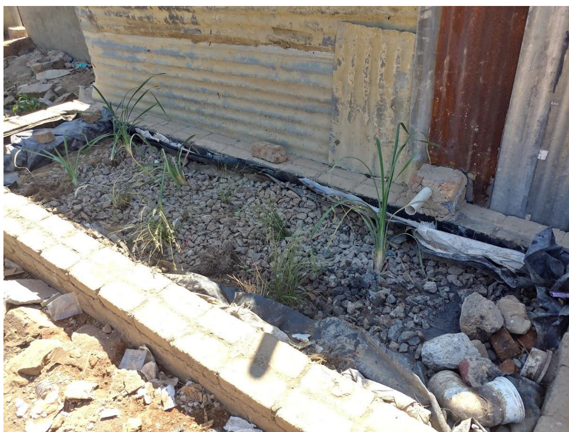
Figure 65: Constructed Wetland 1 showing an informal house that was built on one of its retaining walls with a drain leading into the middle area of the wetland and bypassing the inlet
