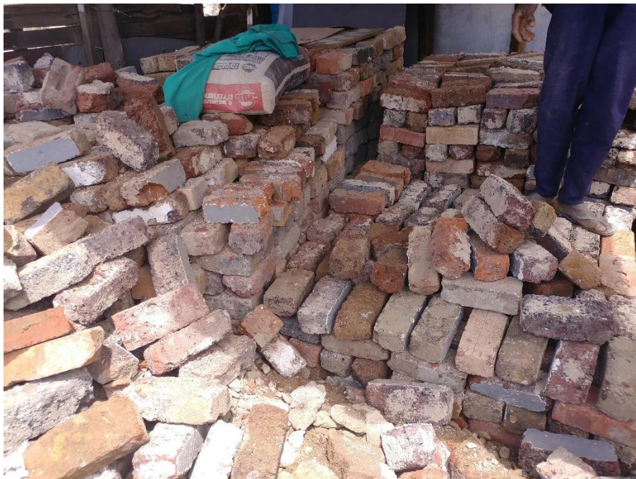
Figure 10: Re-used bricks that were procured from a local supplier in Silvertown, Alexandra for building the containing walls of the constructed wetland
