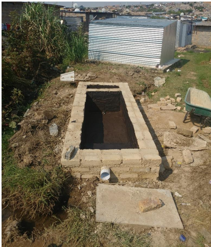
Figure 18: Constructed wetland 2 showing main retaining walls completed and waterproofed
