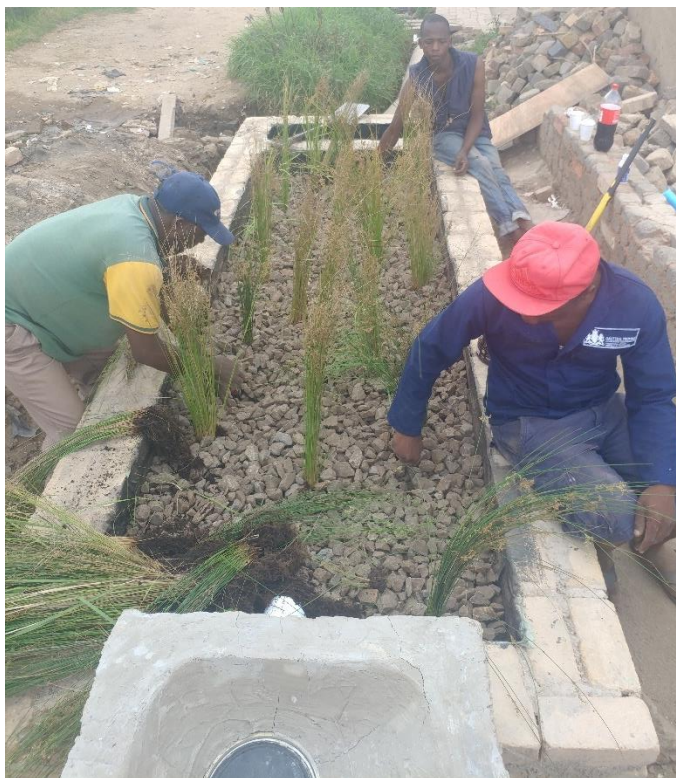
Figure 20: Constructed wetland 1 completed with builders and residents planting reeds
