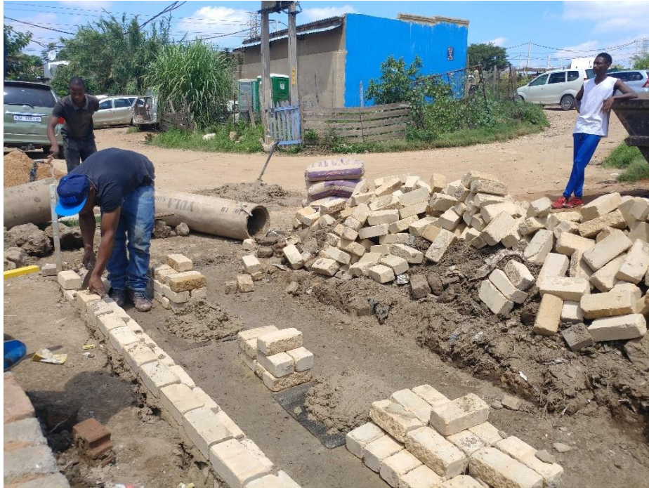
Figure 17: Builders laying foundation and retaining walls for Constructed Wetland 1
