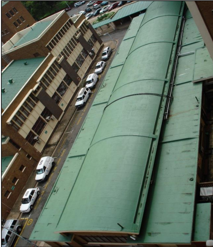
Figure 3. 11: Plan view of roof prior to green roof installation for the Green Roof Pilot Project
