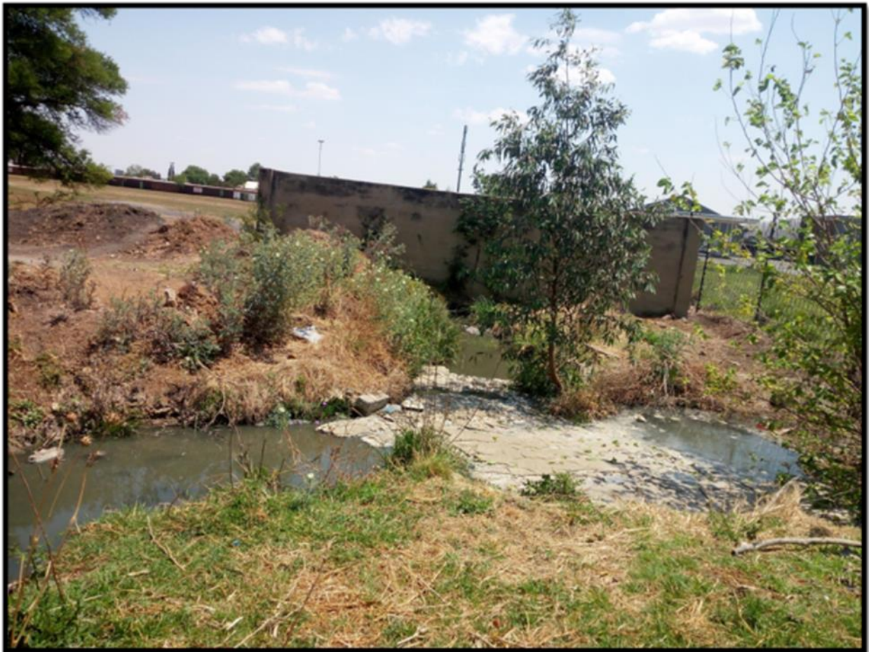
Photo 4.4: Sewage pipe diverted into a stream (source: author's photograph, 18 October, 2019).
