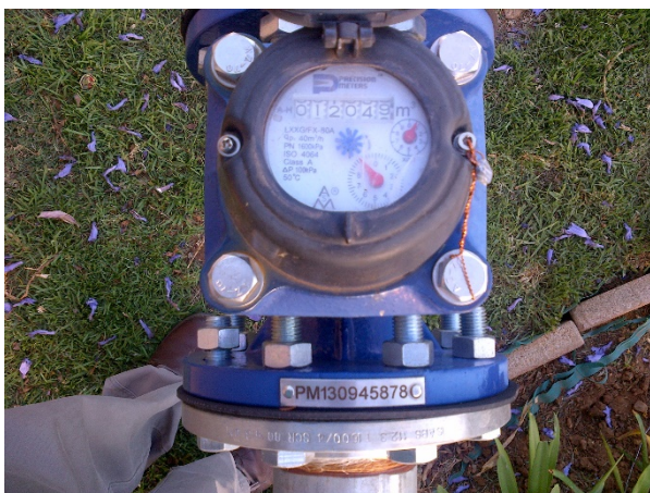
(c) Class A meter for a multi-residential unit, with no pulse output
