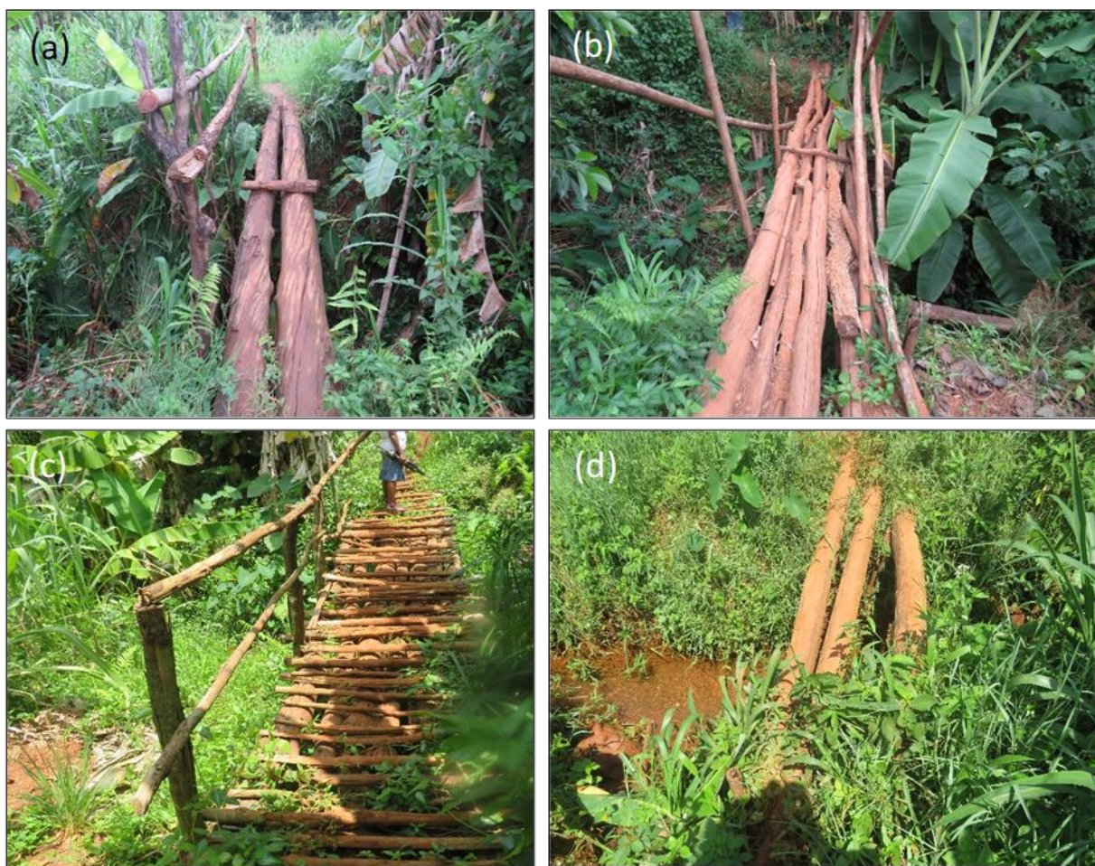
Figure 5.38: Wooden log bridges. (a) Wooden log bridge with supporting side logs that people can hold to assist them when crossing one of the rivers in Rutsate wetland; (b) wooden log bridge with supporting side logs built over a trenches that had developed into a stream in Mareya wetland; (c) log bridge on one of the trenches in Mareya wetland; (d) log bridge built on one of the small streams in Tawarara A wetland (photos: Emmah Mandishona)
