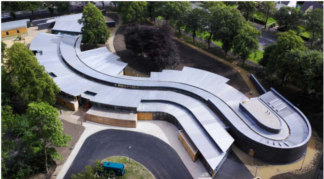
Figure 2.23. Birds-eye view of Hazelwood School. Photo courtesy of Alan Dunlop Architects. https://aasarchitecture.com/2016/09/hazelwood-school-glasgow-alan-dunlop-architect.html/ (accessed 12-12-2019)
