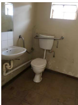
Figure 4.34. Accessible toilet 2 at schools visited. (Author, 2018)
