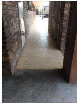
Figure 4.28. Corridors and finishes at schools visited (Author, 2018)
