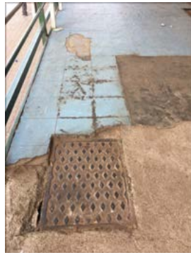
Figure 4.29. Corridors and finishes at schools visited (Author, 2018)
