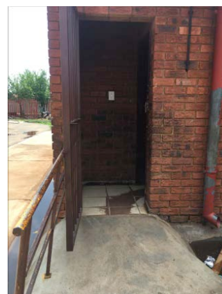
Figure 4.35. Accessible toilet 3 at schools visited. (Author, 2018)
