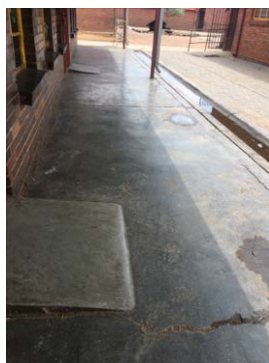
Figure 4.30. Corridors and finishes at schools visited (Author, 2018)
