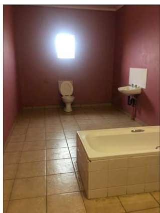
Figure 4.33. Accessible toilet 1 at schools visited. (Author, 2018)
