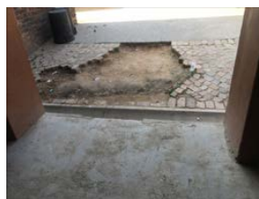
Figure 4.31. Corridors and finishes at schools visited (Author, 2018)
