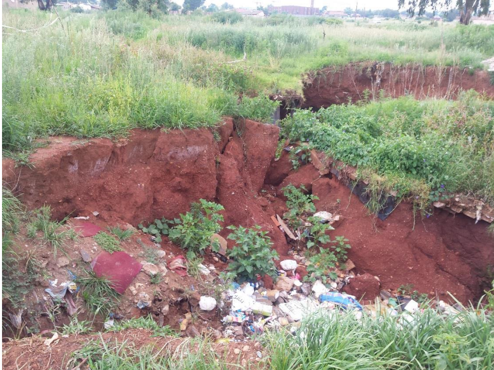
Figure 2: In 2015, a sinkhole opened in the Thembelihle informal settlement, attributable to the presence of dolomite in the area. Photo by author. Date: 17/01/2017
