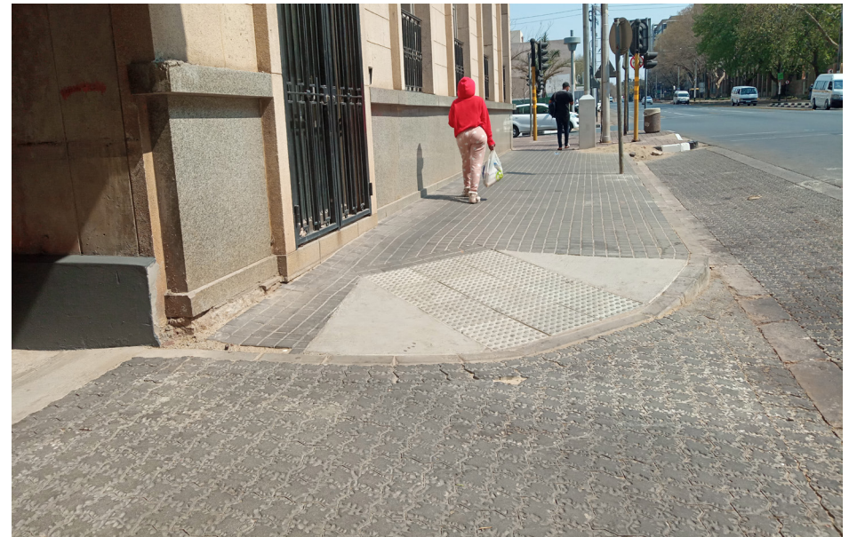
Fig 26: Gently sloped ramp across driveway on sidewalk 2a
