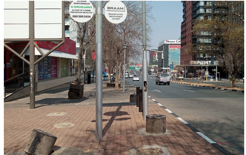
Fig 23: Protrusions along sidewalk 4b
