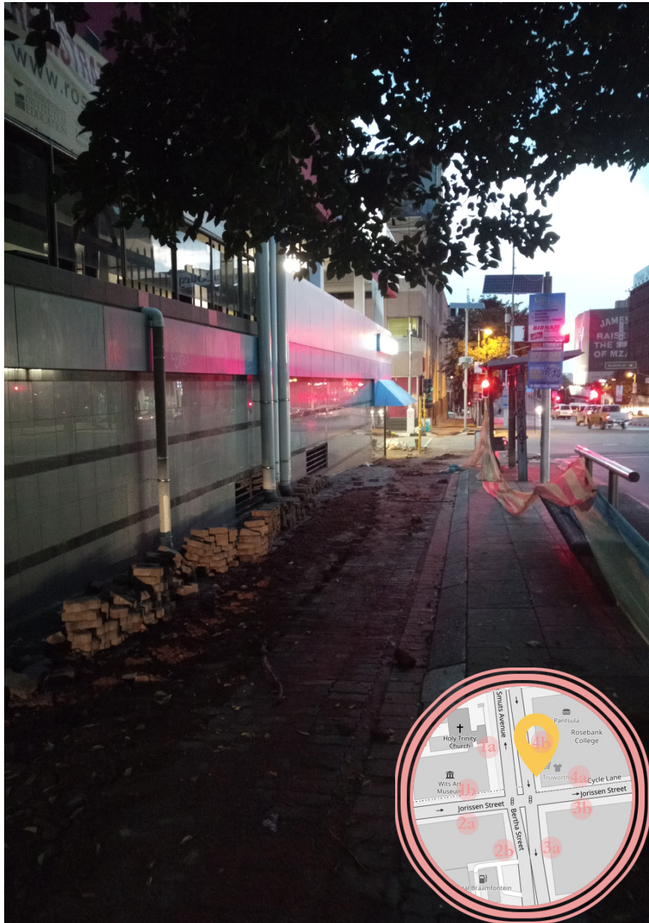
Fig 31: Sidewalk 4b during construction works
