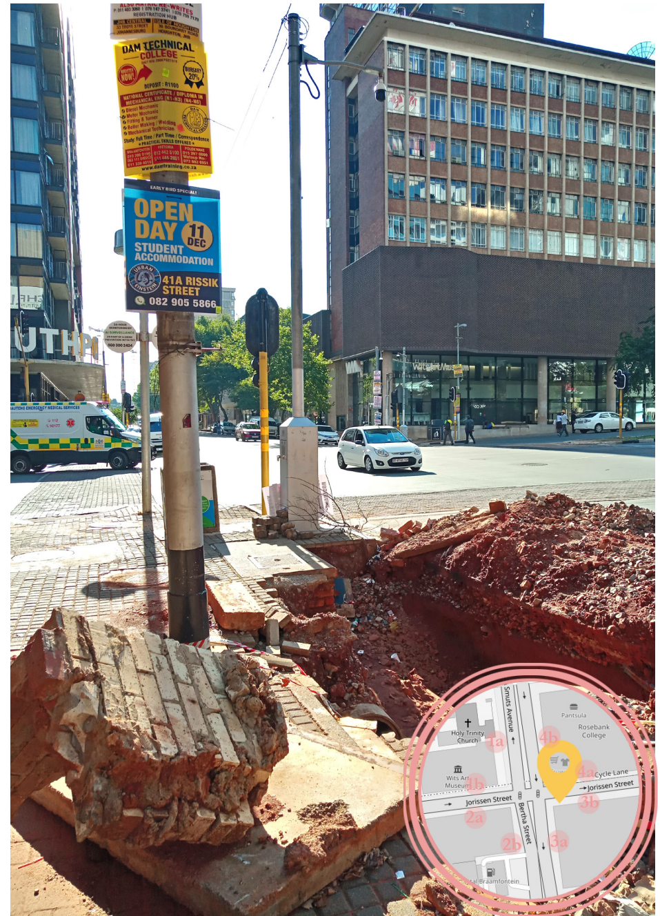
Fig 30: Sidewalk 4a during construction works
