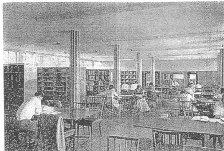
Fig. 4.24 John Moffat Building: library and foyer-exhibition area.
