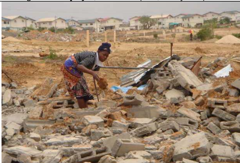
Plate 6-7: Cambamba I – Municipio do Kilamba Kiaxi, demolition and displacement. (Anonymous)
