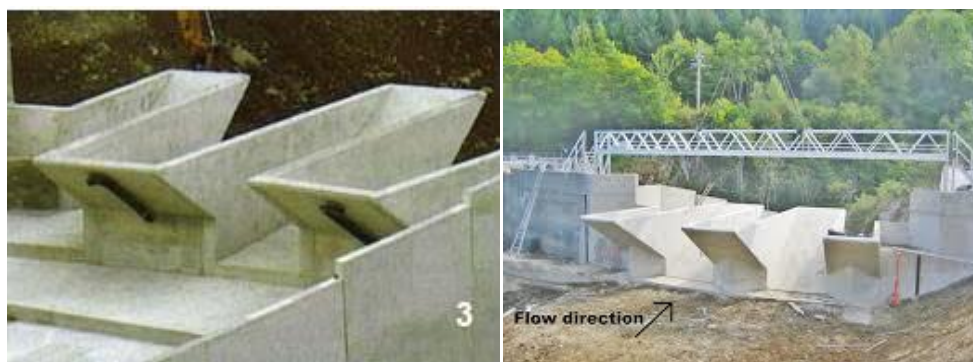
Figure 2.19: Goulors dam in France (Anon., n.d.)
