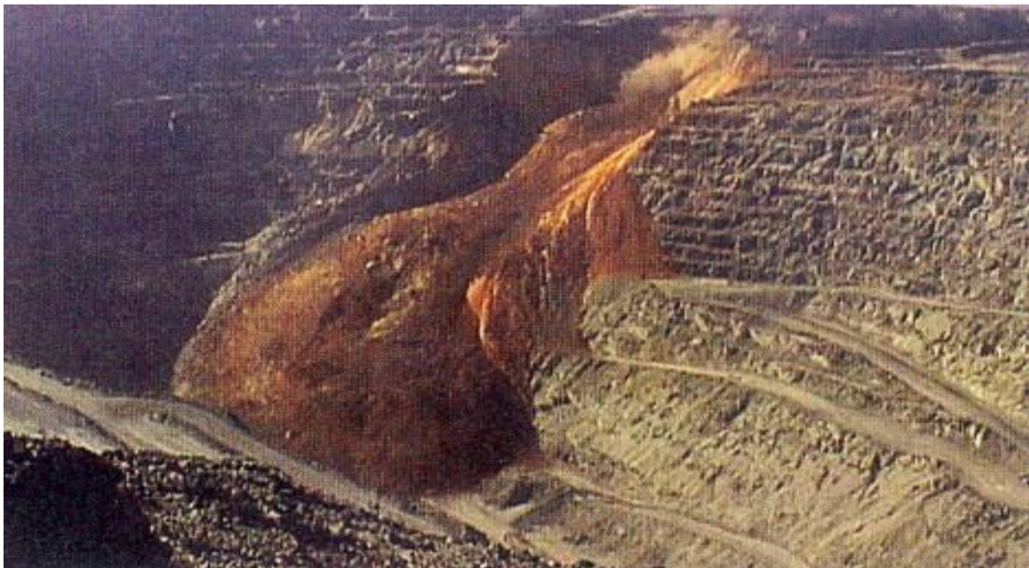
Figure 2.10: Large-scale wedge failure disrupting the entire mine slope (After Lorig, et al. 2009).
