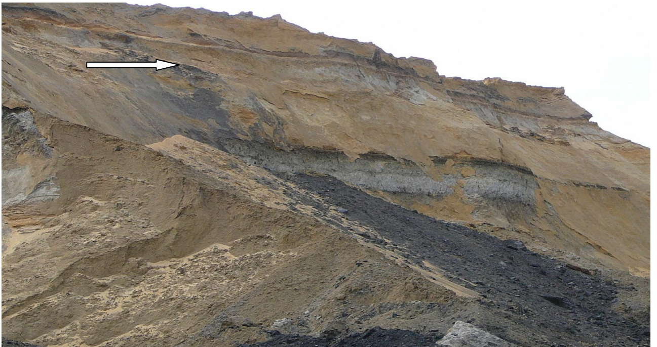
Figure 2.4: Unstable sand overburden at New Vaal Open-cast coal mine.
