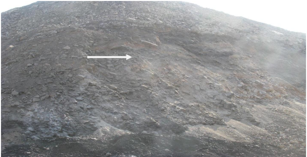
Figure 1.5: Failed low-wall resulting from undercutting at Kleinkopje open-cast coal mine.
