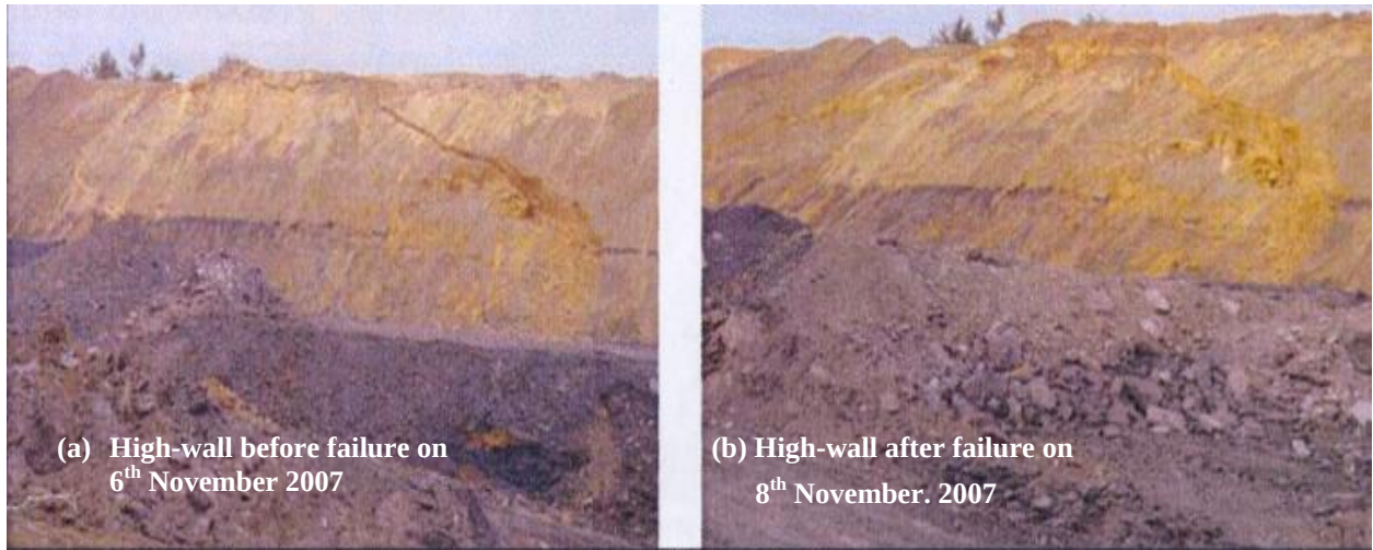
Figure 4.14: High-wall before and after failure (Zindela, 2008).
