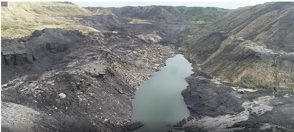
Figure 20: Drone image of the complete interburden failure of the highwall in Ramp 2-4.
