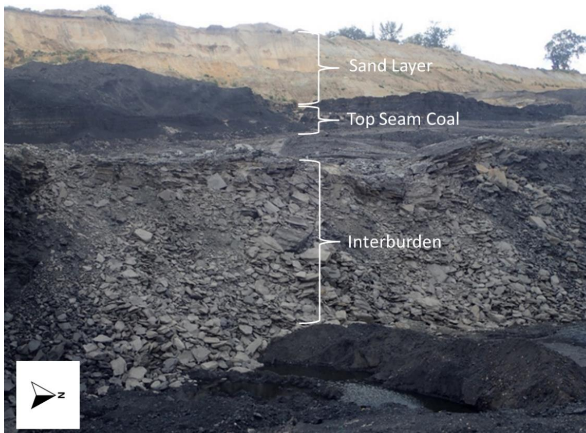
Figure 17: A second interburden failure that took place on the highwall of Ramp 2-4.
