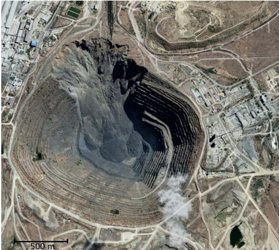
Figure 9: Slope failure at Palabora copper mine (Woo et al., 2012).
