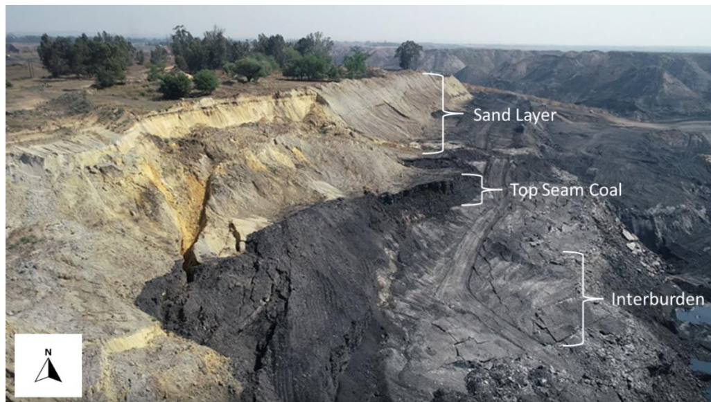
Figure 15: Ramp 2-4 highwall failure on 22 October 2020.
