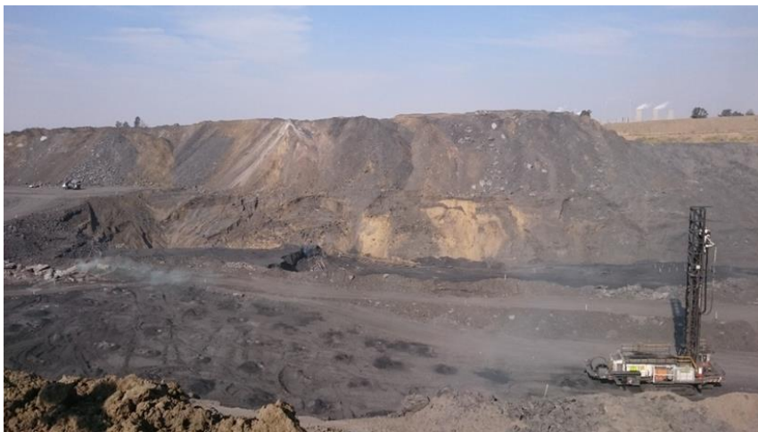
Figure 11: Ramp 19 low wall failure that occurred on 18 August 2016.
