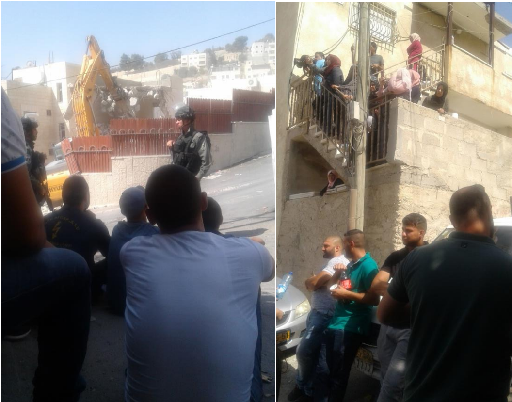
Figure 8 Israeli forces stand between the community and the bulldozer as it completes the demolition. All residents can do now is watch
