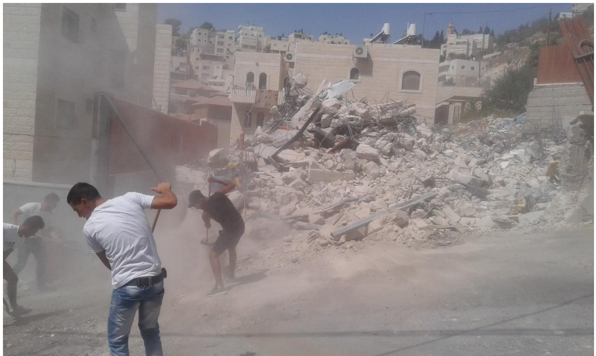
Figure 11 Cleaning the rubble after the demolition
