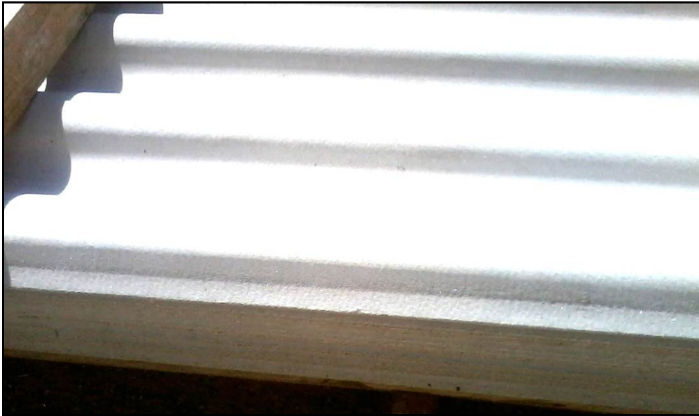
Figure 6.53: Corrugated sheets, 3% kaolin replacing cement, with downturns orientated in the direction of highest incidence of solar radiation, no cracks observed.
