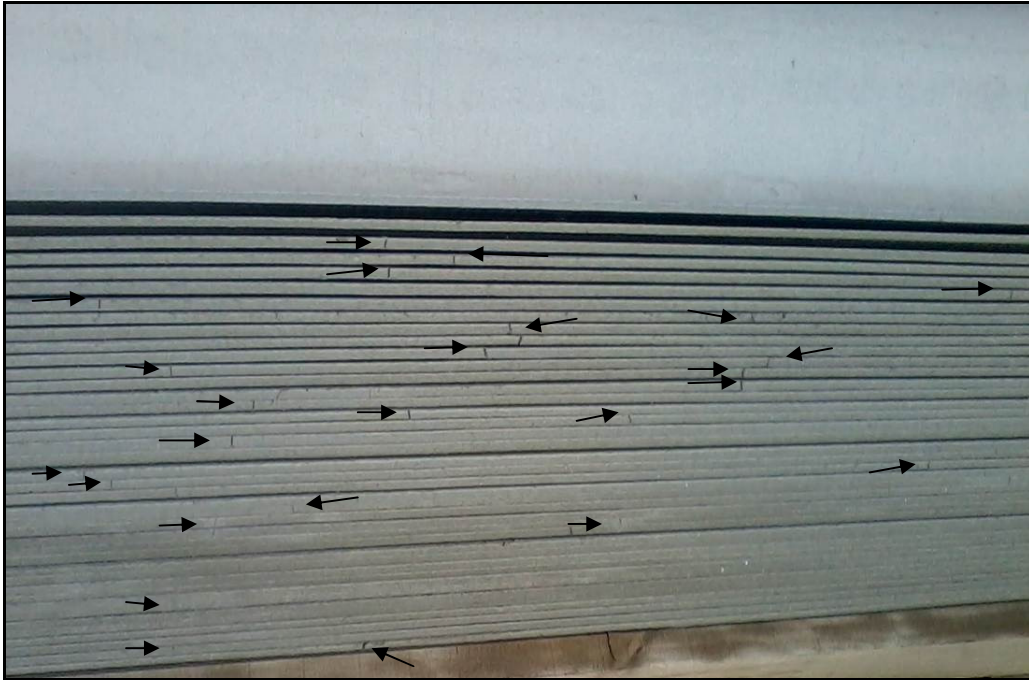
Figure 6.35: Kaolin modified corrugated sheets cured outside, without plastic wrapping, showed wide edge cracks after 30 days curing.
